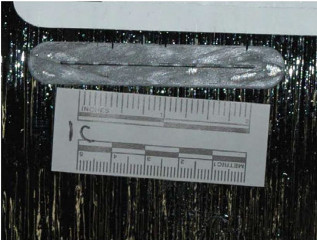
Figure A5: Tank 1C, Longitudinal Flaw Direction
