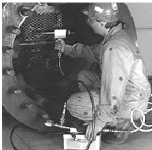
Fig. 3 Typical Installation of Mechanical Fit Tube Plugs (©2006 Photo courtesy of EST Group Inc., used with permission.)
