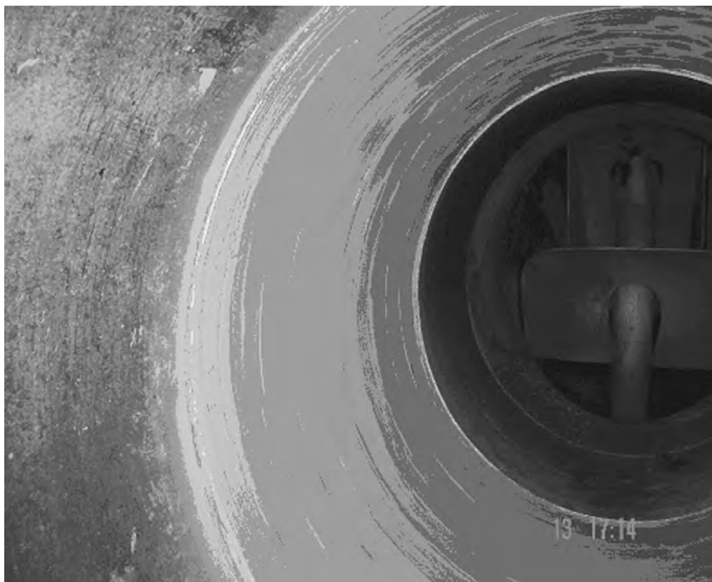
Fig. 1 Structural Liner in Raw Water System
