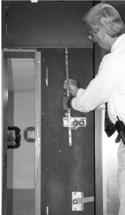
Fig. 1.3.4(d) Opening Hoistway Door by Hand (Not Possible on Some Elevators)
