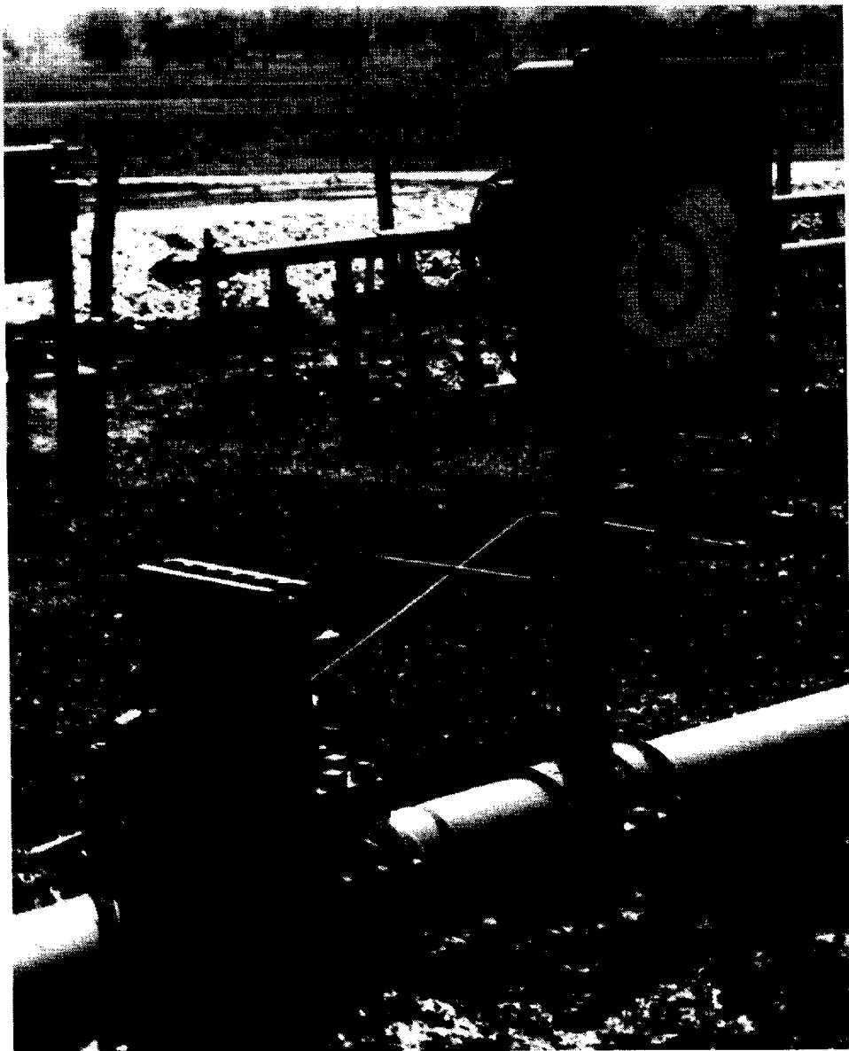
Figure 111—Small pipes, valves and fittings connect gas meter to meter run. Flanged device at lower left contains orifice plate; fitting above permits plate installation and removal.
