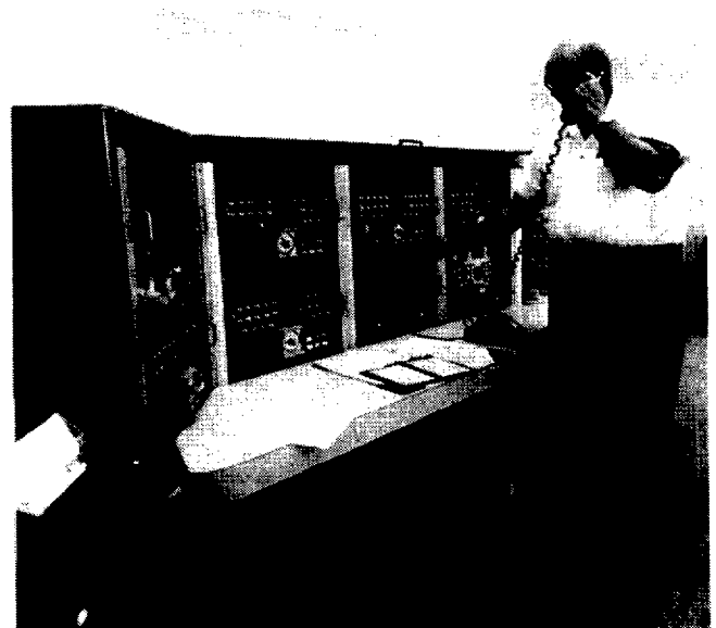
Figure 72—The master station controls and monitors operations through a communication system of satellites and remote control panels connected to the end devices.
