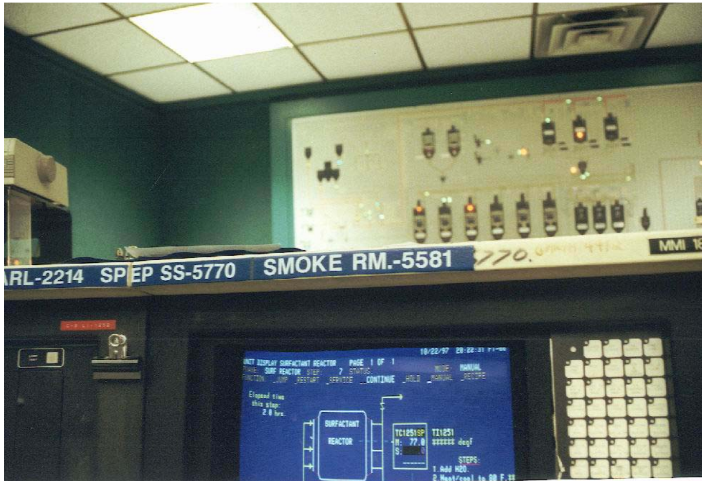
Figure 9—Operator's View of Wall Displays is Obstructed by DCS Console
