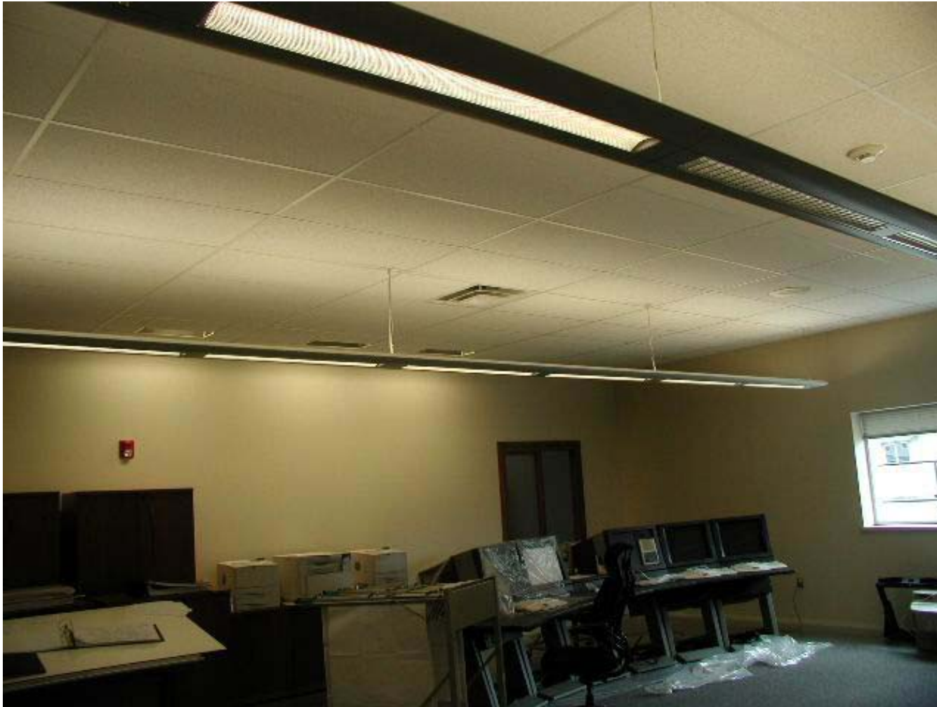
Figure 8—Indirect Lighting Applications Can Control Reflected Glare
