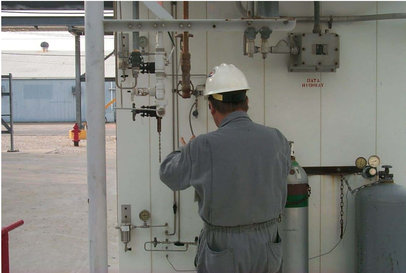
Figure 13—Avoid Head Knockers Adjacent to Analyzer Building Work Area
