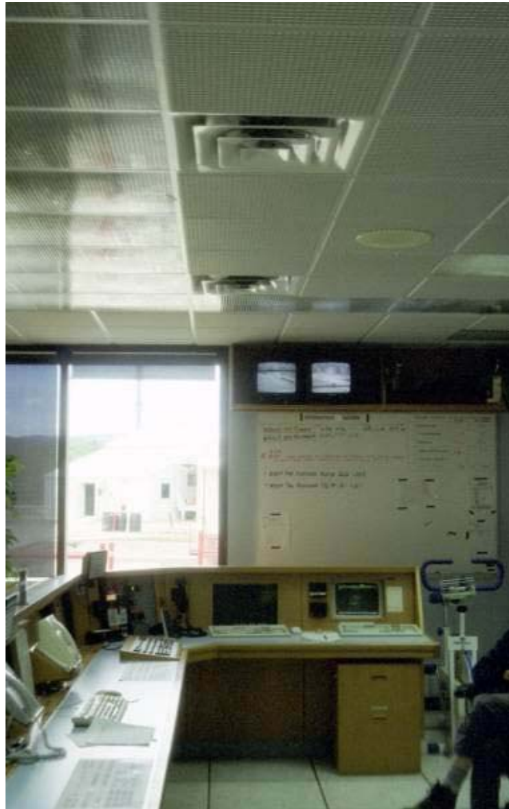
Figure 12—Security Monitors Mounted Above and Behind the Control Room Operator's Position
