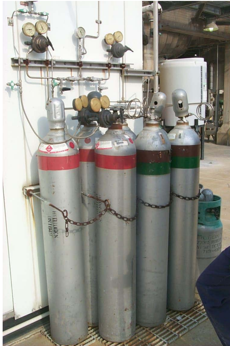
Figure 15—Gas Bottle Access is Obstructed by Bottle Arrangement
