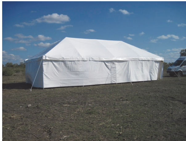
Figure A-9—Guy Wire Locations at Corners and Middle of Long Side
