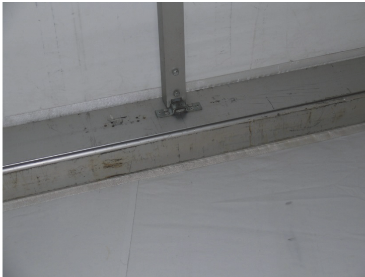
Figure A-20—Connection of Purlin to Frame
