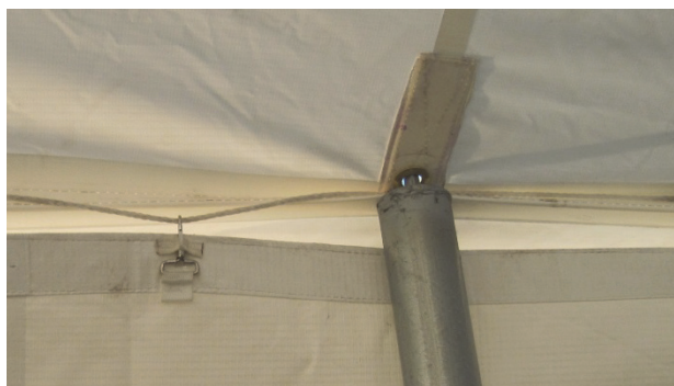
Figure A-3—Detail of Fabric, Rope, and Pole Connections
