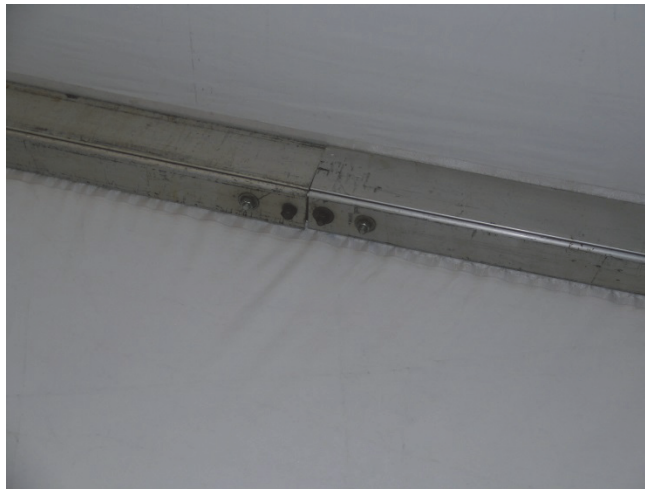
Figure A-18—Frame Splice Develops Partial Moment Capacity
