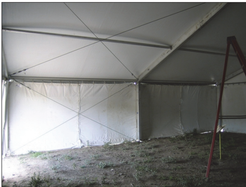
Figure A-16—Interior of Rigid Frame Tent
