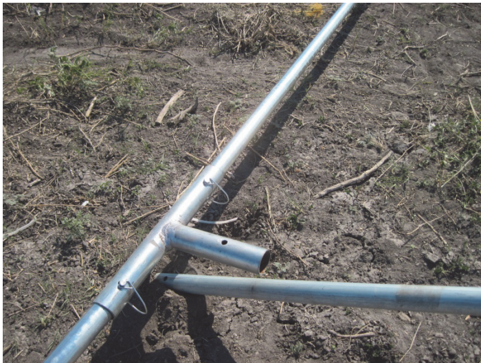
Figure A-6—Connection Hub at Center of Long Wall
