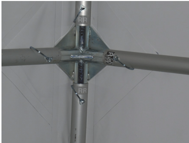
Figure A-27—Center Hub Connector
