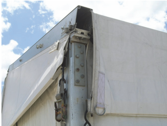
Figure A-17—End of Framing Member Showing Extrusion Shape and Connection
