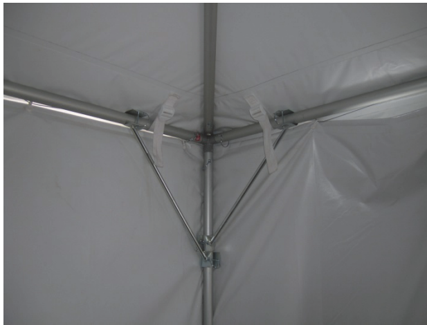
Figure A-24—Tubular Bracing at Corners
