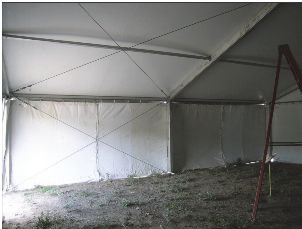
Figure 56. Internal View of Moment Framed Tent Showing Frames and Cross Bracing
