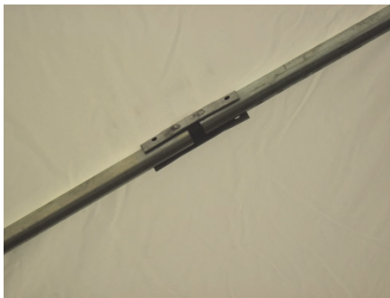
Figure A-5—Detail of Rafter Hinge (Cotter Pins still need to be installed.)
