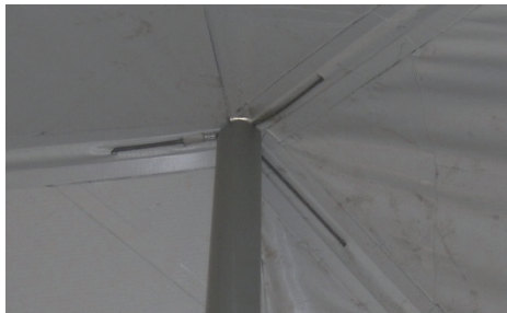
Figure A-13—Top of Interior Pole Showing Cables Embedded in Fabric
