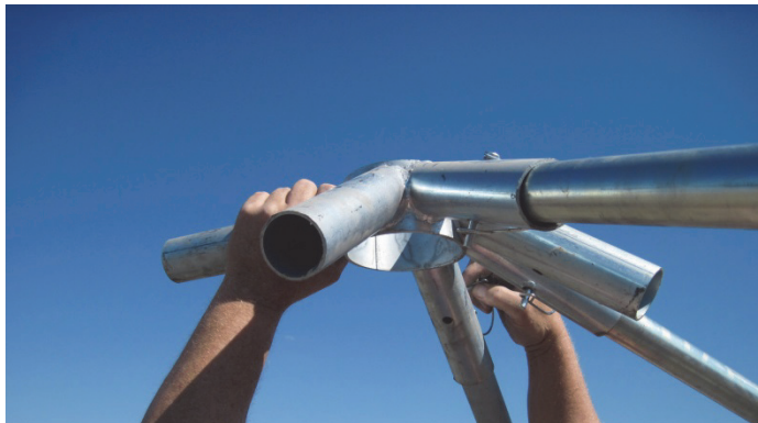
Figure A-7—Connection Hub at Top of Gable End
