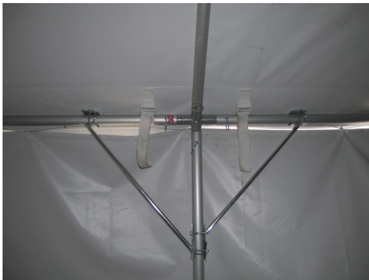
Figure A-25—Tubular Bracing at Sides
