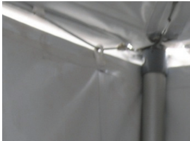
Figure A-14—Plastic Clips Securing Side Panels to Perimeter Rope
