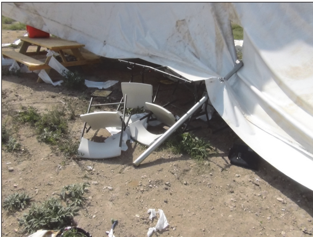
Figure 89. Damage to Pole Tent and Displacement of Table and Chairs
