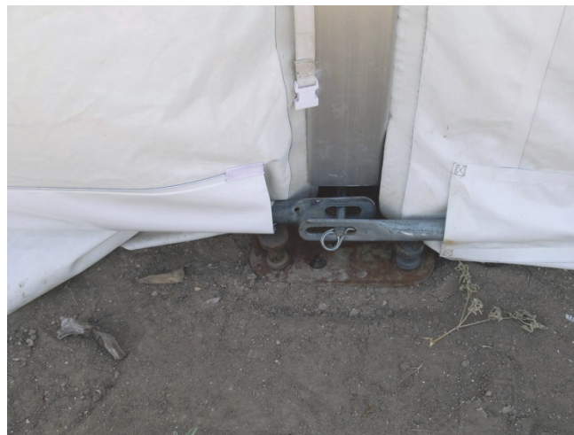
Figure A-21—Method Used for Securing the Bottom of the Wall Fabric
