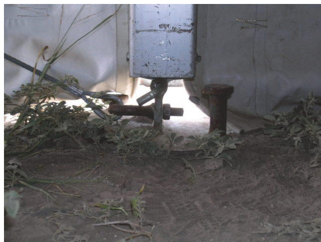
Figure A-19—Frame Base Plate Showing Cable Connection
