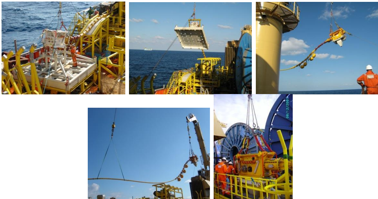
Figure 8—Illustration of Impact of MBR/ABR During Various Stages of Installation
