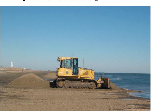
Figure 5.30 Sediment Relocation using Front-End Loader
