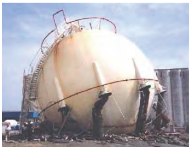
Figure 5—Failure of Sphere Legs Due to CUF
