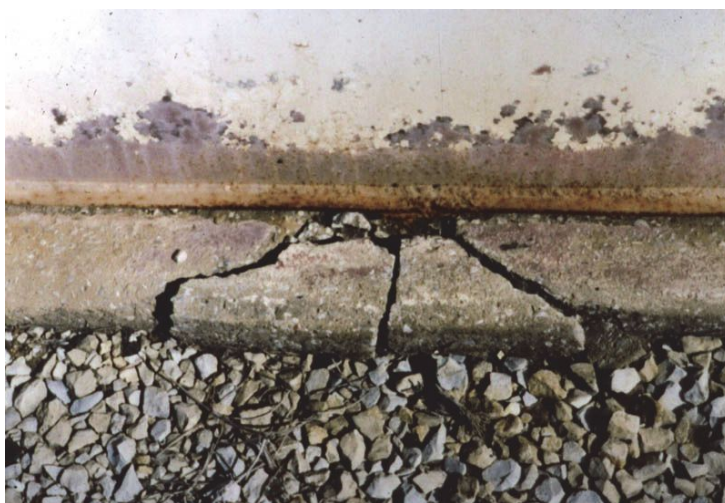
Figure 34—Failure of Concrete Ringwall
