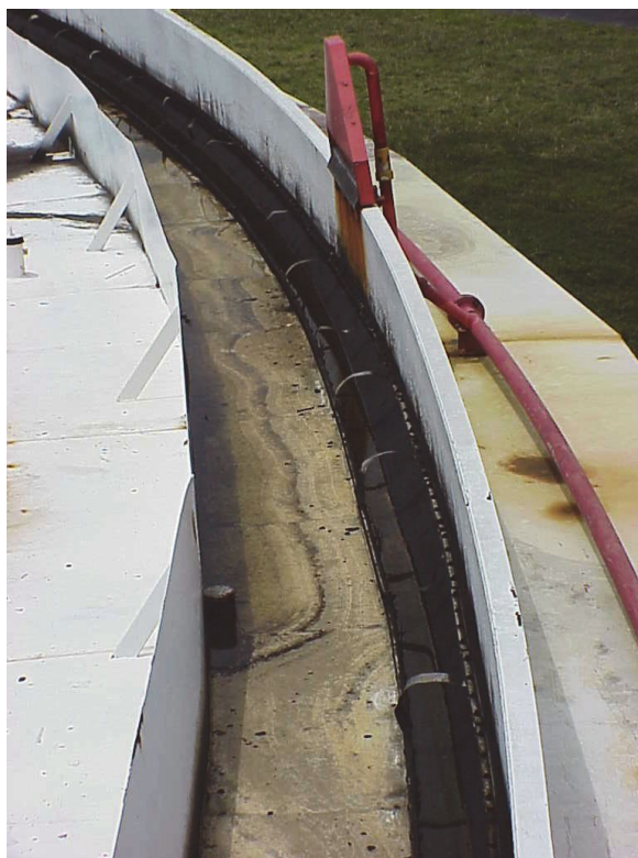
Figure 46—Deterioration of Floating-roof Seal
