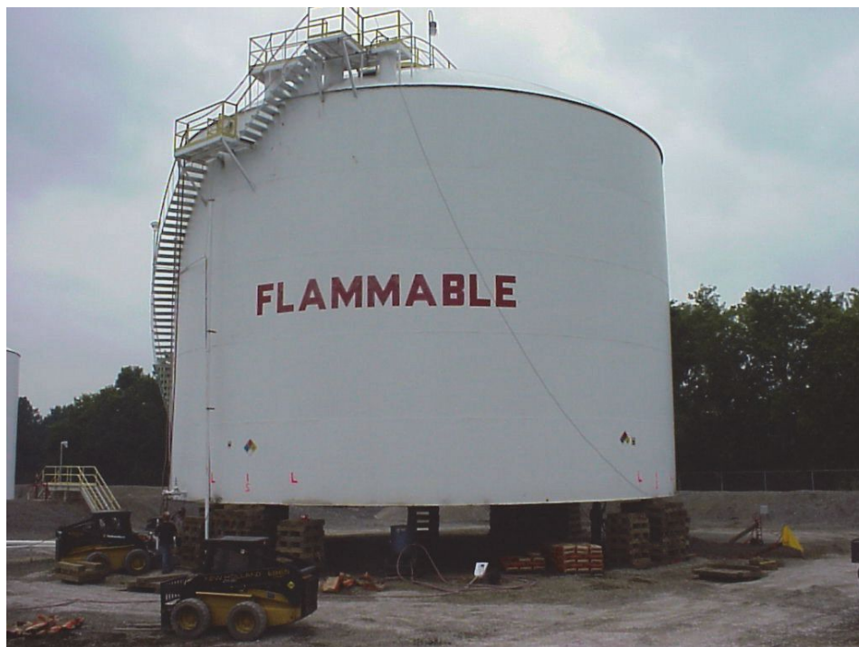
Figure 69—Tank Jacked Up for Repairing Pad
