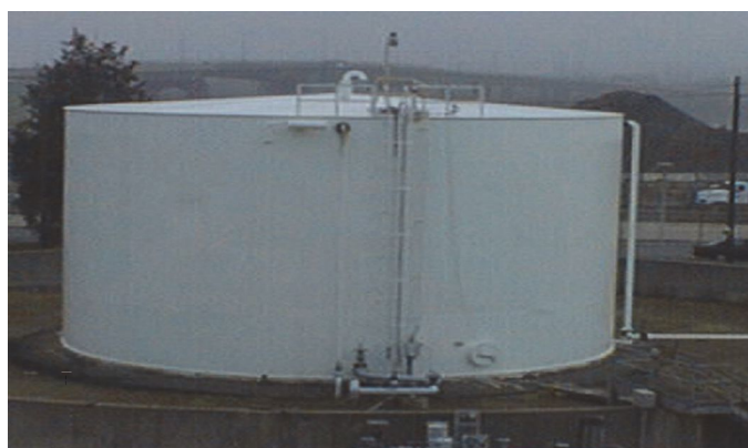
Figure 1—Cone Roof Tank
