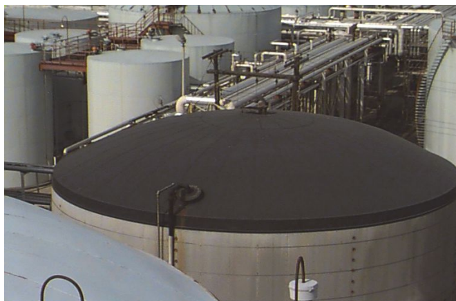
Figure 4—Self-supporting Dome Roof Tank
