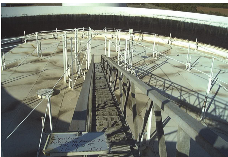
Figure 5—Pan Type Floating-roof Tank
