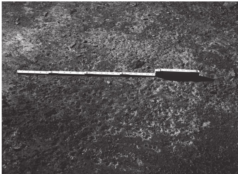
Figure 54—Example of Extensive Corrosion of a Tank Bottom
