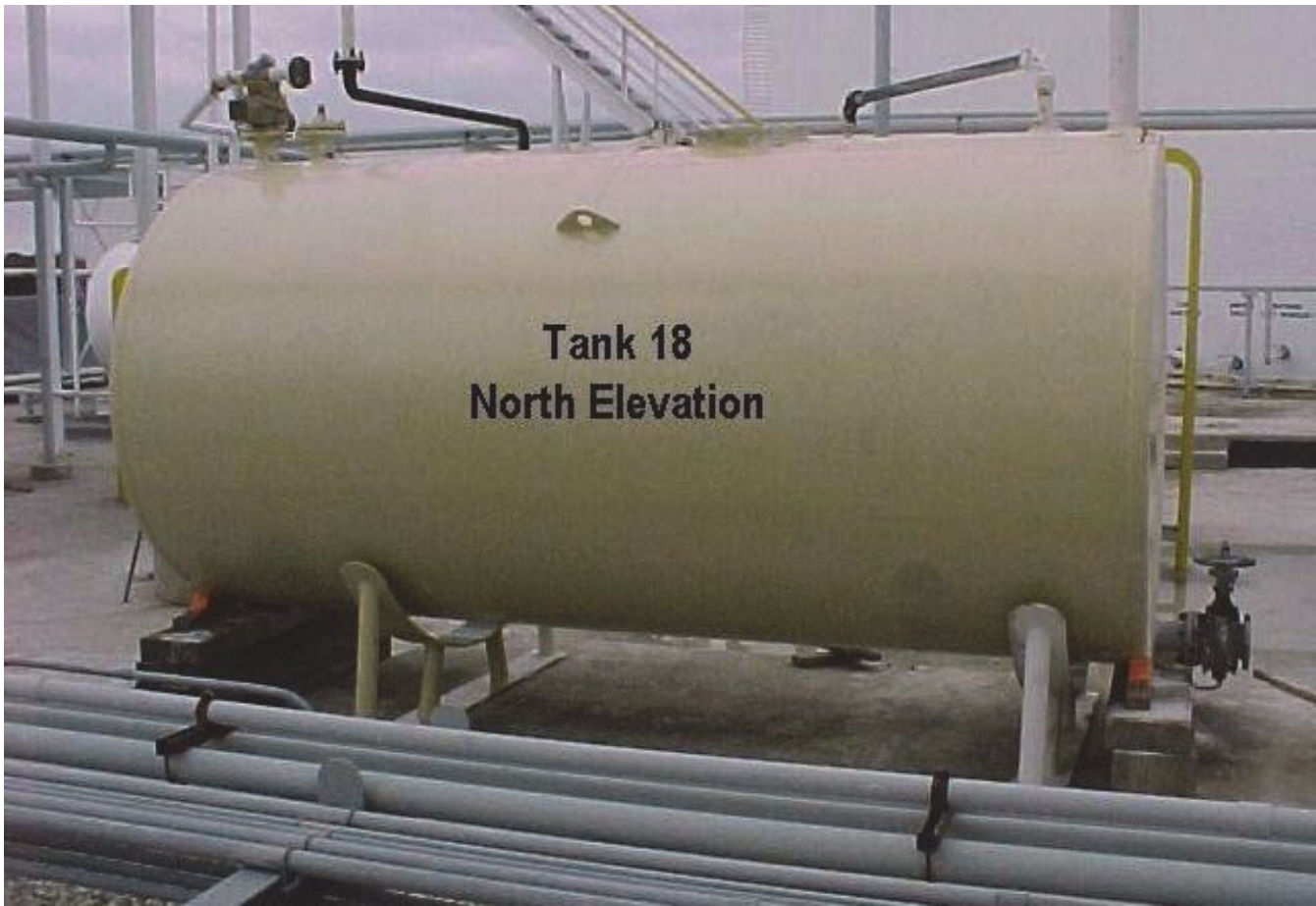
Figure 20—Welded Horizontal Tank Supported on Saddles
