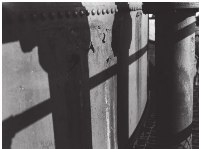
Figure 56—External View of Erosion-corrosion Completely Penetrating a Tank Shell
