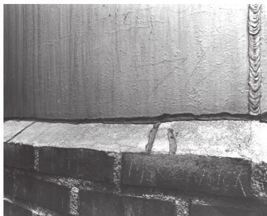
Figure 28—Foundation Seal
