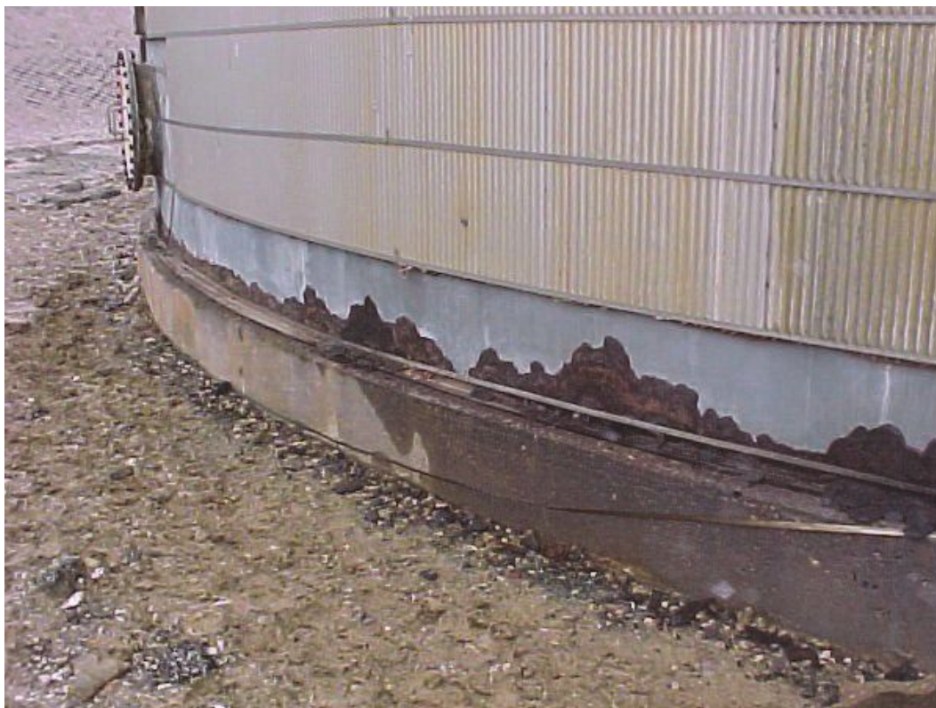
Figure 37—Corrosion Under Insulation
