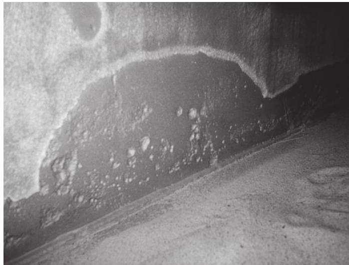
Figure 55—Shell-to-bottom Weld Corrosion
