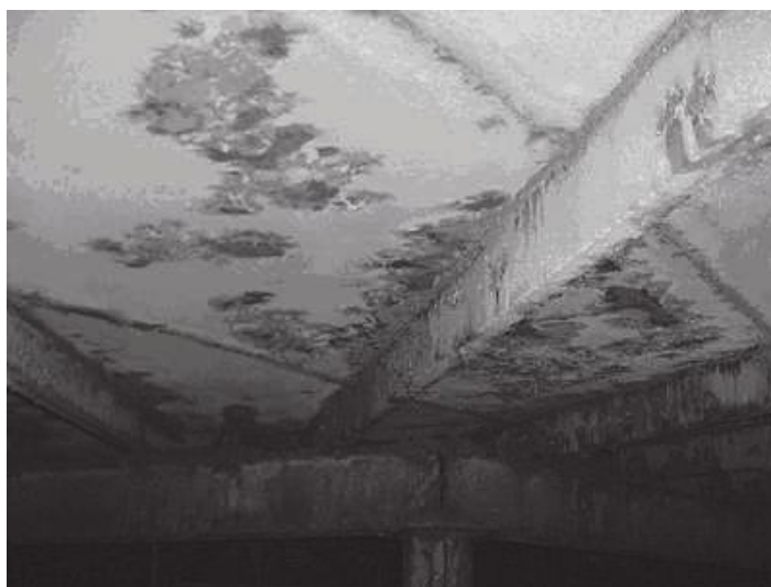
Figure 58—Internal Corrosion on Rafters and Roof Plates
