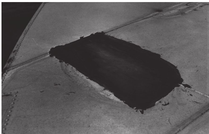
Figure 67—Temporary “Soft Patch” Over Leak in Tank Roof
