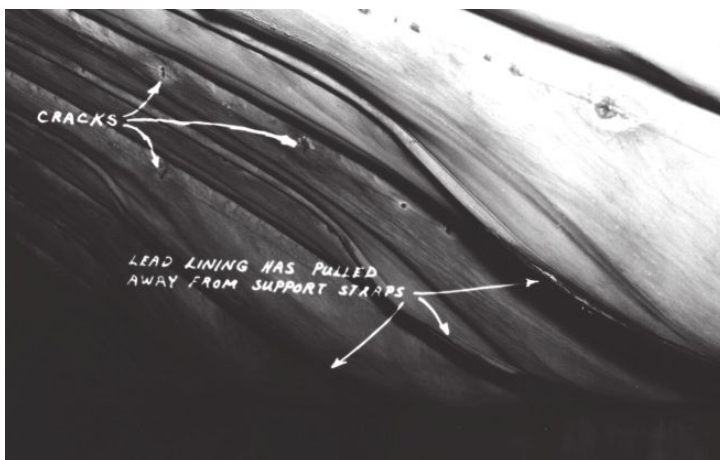
Figure 57—Deterioration of Lining on Roof of Tank Caused by Leaks in Lining
