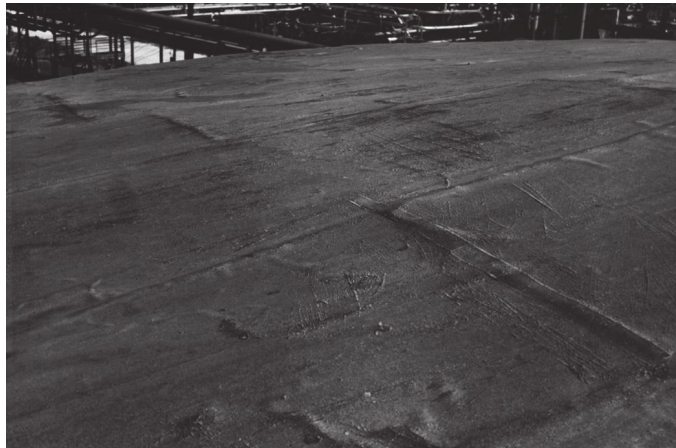
Figure 68—Mastic Roof Coating
