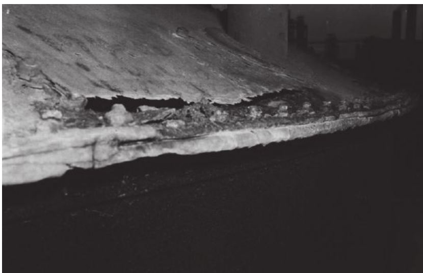
Figure 45—Example of Severe Corrosion of Tank Roof
