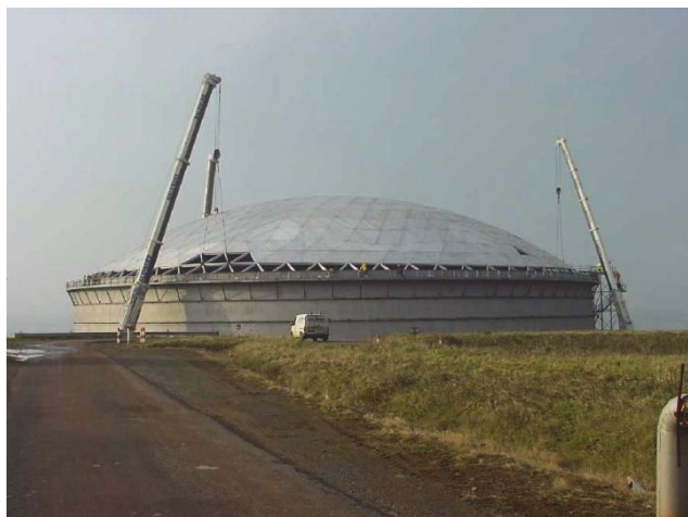
Figure 3—Geodesic Dome Roof Tank
