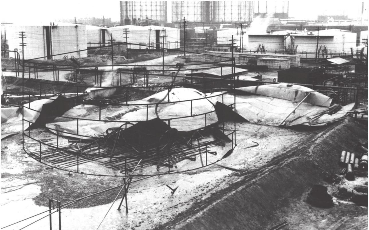
Figure 30—Extensive Destruction from Instantaneous Failure
