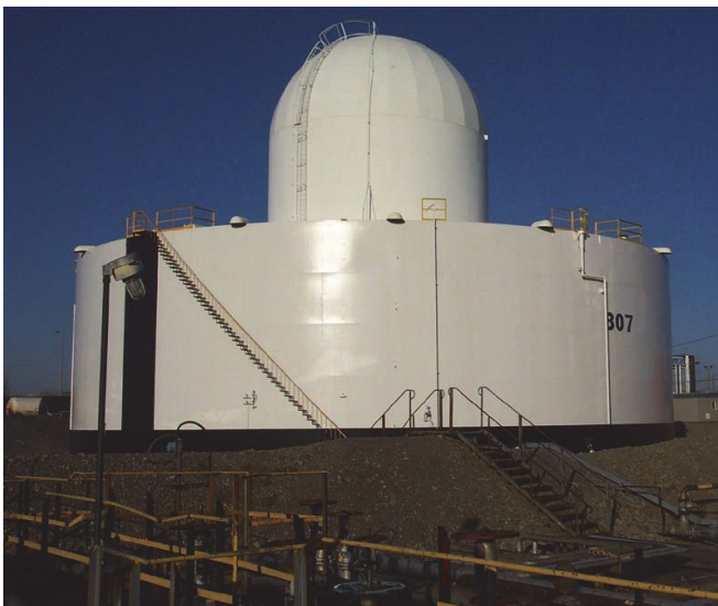
Figure 17—Tank with Vapor Dome Roof
