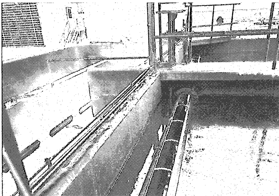
Figure 10—General Arrangement of Rotatable Slotted-Pipe Skimmer
