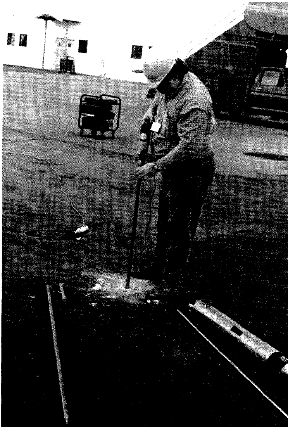
Figure 19. Drilling to Get Access to Pipe for Acoustic Emissions System
