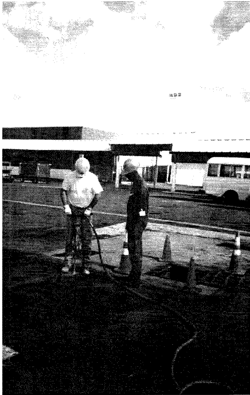
Figure 8. Drilling to Install Tracer Ports
