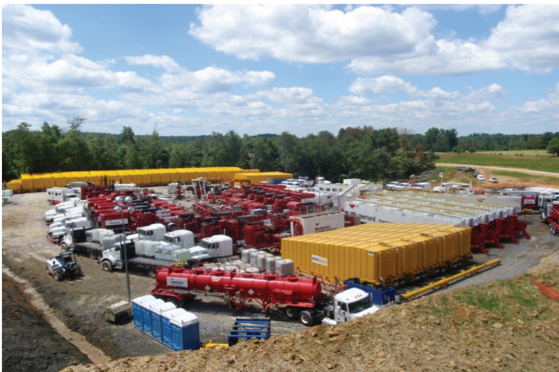
Figure 4—Hydraulic Fracturing Well Site for a Marcellus Shale Well
