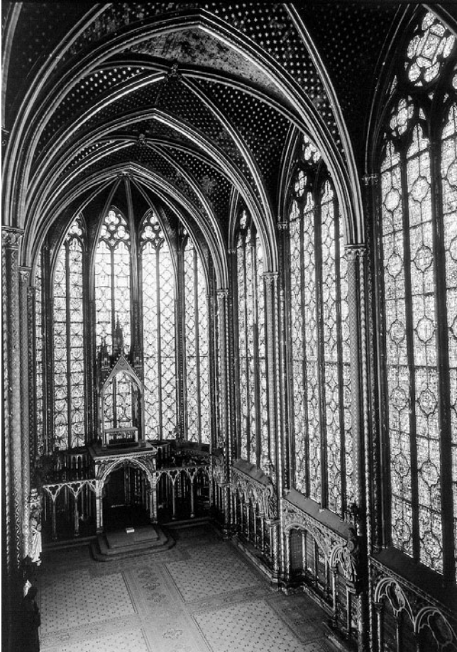
Interior of Sainte-Chapelle, Paris. The stained-glass windows of the Sainte-Chapelle (1246–1248) are a fine example of the vibrancy of Gothic art. The pointed arches and ribbed vaulting of the Gothic style can also be seen clearly. (Giraudon/Art Resource, NY)
