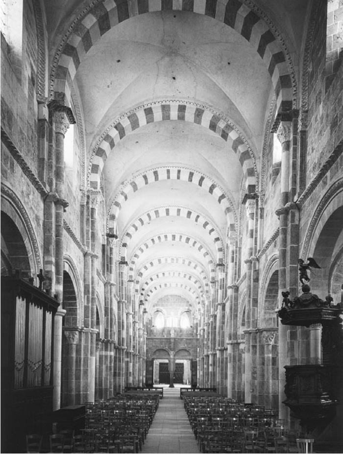
Basilica de la Madeleine, Vezelay. There were many local variations on the Romanesque and Gothic styles of architecture. In this example, the abbey of La Madeliene in Vezelay (1104), the barrel-vault of the nave was replaced by a new style that utilized a groined-vault and transverse arches. The redistribution of weight and stress that this involved made possible the introduction of more windows, thus creating a more open and airy effect. (Scala/Art Resource, NY)
