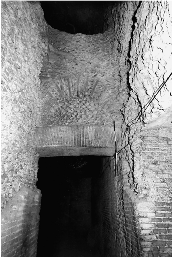
41. Room 27A: Overview to the south, with Neronian Type E facing to the west (right) and the scar below the lintel where the original jamb spur was cut away.
