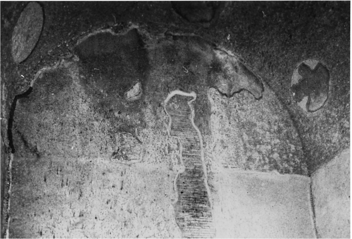
56. Room 45: The lunette of the east end (detail of Fig. 52). At the top, the dark patch left of center is the only visible remnant of the original Neronian fresco decoration. The diagonal seam at the top of this decoration reveals the strike of the Neronian phase 1 pitched roof. The lighter plaster above that seam, running up to the intrados of the vault, is the fill-in decoration from when the Neronian phase 2 vault exposed this portion of the wall for the first time (the stippled area in Fig. 53.2). The grotto decoration scheme (all other decoration visible in this photo) was then applied on top of these two phases of frescoes.
