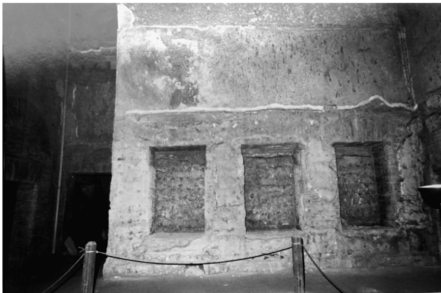
57. Room 45: Elevation photo of the north side.
