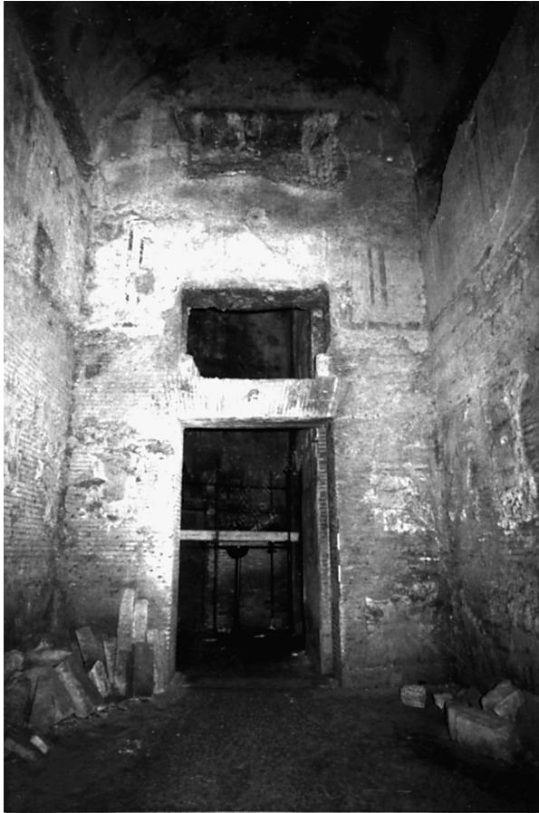
14. Room 76: Overview to the north. The pre-Neronian skylight is at the top of the photo, filled in; the window just above the door is a post-Neronian modification.
