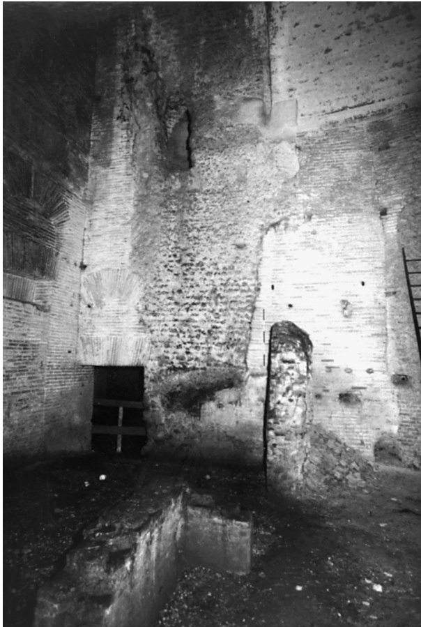
58. Room 51: East side, north half. L–R: south side of Room 45; Type E masonry with the doorway to Room 69; scar where Room 69 was trimmed off to make way for Room 51; patch of Type G masonry (Neronian phase 2), with the meter on it and the Type J cross wall in front of it; Type X facing (right edge of photo, just left of the ladder) showing from behind the Type G applied on top of it.
