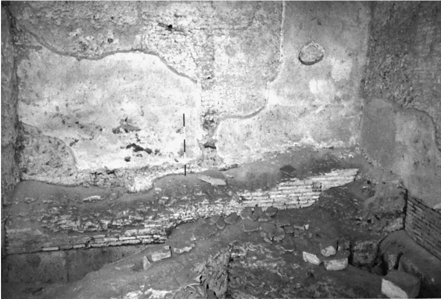
18. Room 54: Overview to the south, showing all four phases in Figure 16. At the bottom center there is the distantly pre-Neronian oblique room, cut off by the Type B masonry, whose ashlar foundation and brickwork appear behind it. At the right end of the Type B wall, the Type Y material appears, addorsed to the front side of the Type B. At the right side of the photo the Neronian Type E west side wall abuts the Type Y from the north. Type C forms the whole back wall, unfaced throughout because it was cast against the standing Type B. The Type B was trimmed below Neronian floor level in Neronian phase 1 (cf. Fig. 17.5).
