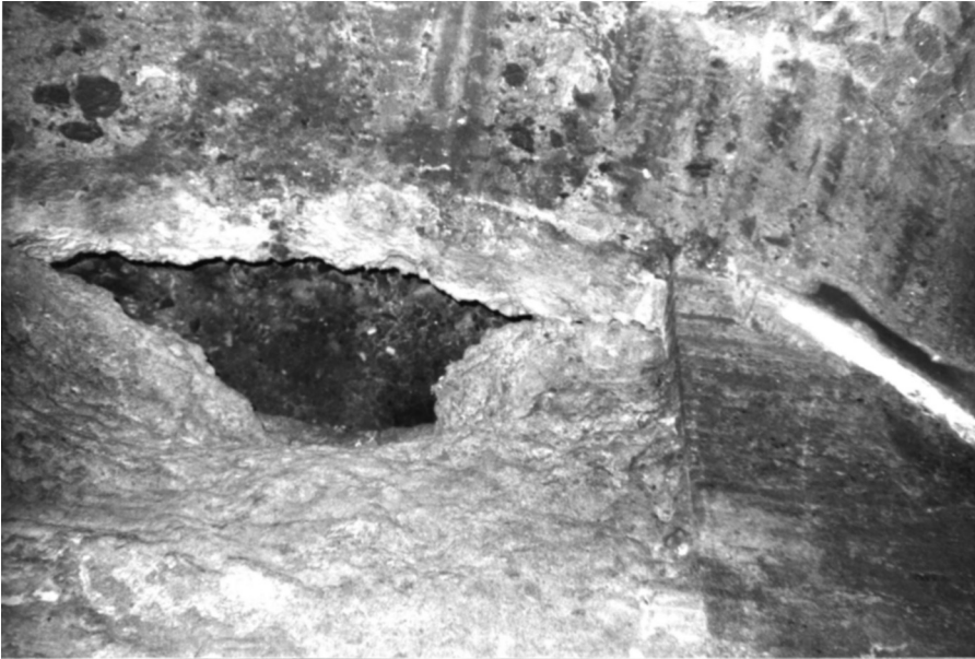
46. Room 40: The small skylight in the south end lunette. The Neronian phase 1 Type E facing forms both the wall surface and vertical sides of the window (right).
