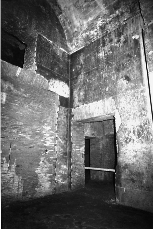
27. Room 116: Overview from southeast to northwest. The window at the left edge is the hypaethraeum , with Trajanic Type M fill in the sellarium doorway below it. The open doorway to the right leads to Corridor 96.
