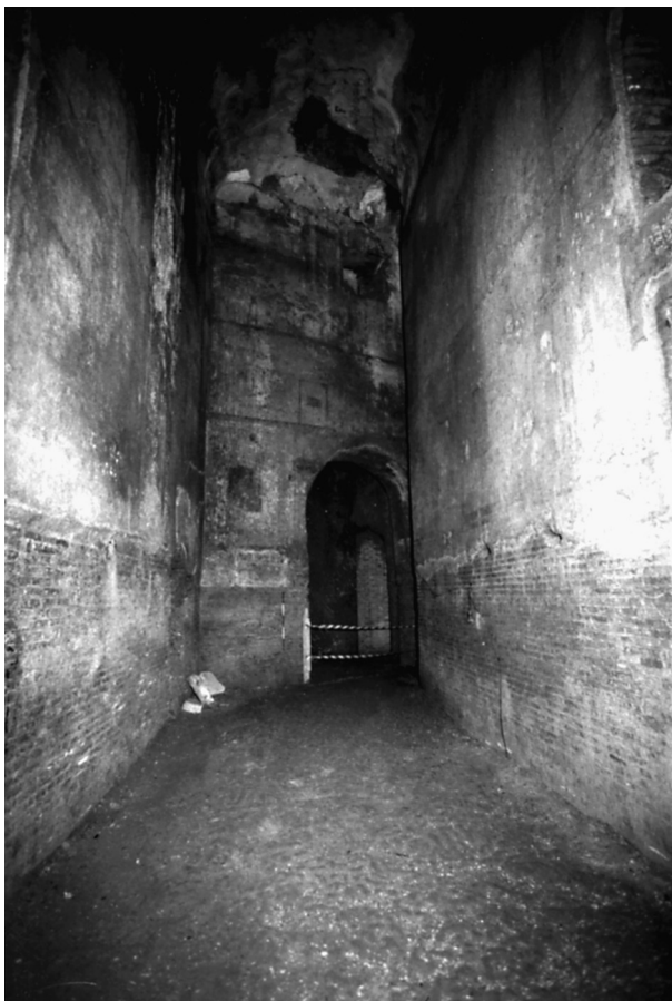
8. Corridor 79: View of the eastern straight section, looking east toward the arched doorway into Room 84 (Type D, with the lunette cut out to raise the lintel to the Neronian level).
