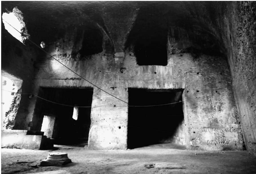
38. The south façade of the West Block in the area of Corridor 22 (L) and Room 24 (R).
