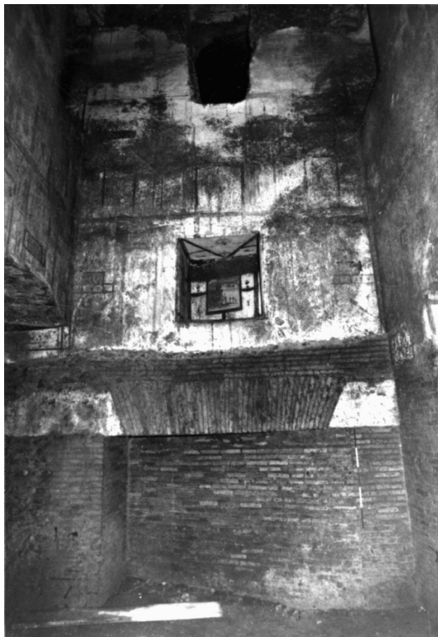
10. Room 85: Overview to the southwest. The small window at the top is post-Neronian. The Type D doorway appears at the bottom, with travertine imposts for the flat arch lintel, filled in with Neronian Type F masonry of the east side of Room 83. The hypoethraeum above it was filled with Type F too, forming a small niche.
