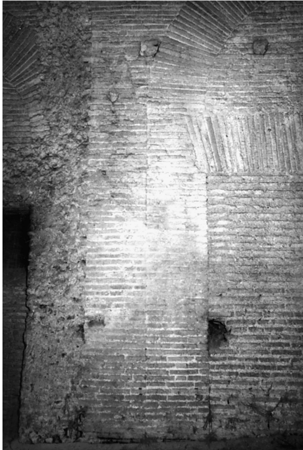
65. Room 51: Detail of the west edge of the apse (cf. Fig. 62, left of center). L–R: the opening of d50.51S (dark), with crude phase 2 tiles completing the original phase 1 half-round relieving arch; scar from the razed phase 1 cross wall, forming the right (north) jamb of d50.51S; phase 1 wall fabric bonding to the core concrete of the cross wall (at the top, the seam left when the flat arch lintel from the large phase 1 doorway was removed); phase 2 wall fabric, forming the left (south) jamb of d50.51N, from which the phase 2 flat and half-round relieving arches spring; late fill in d50.51N.
