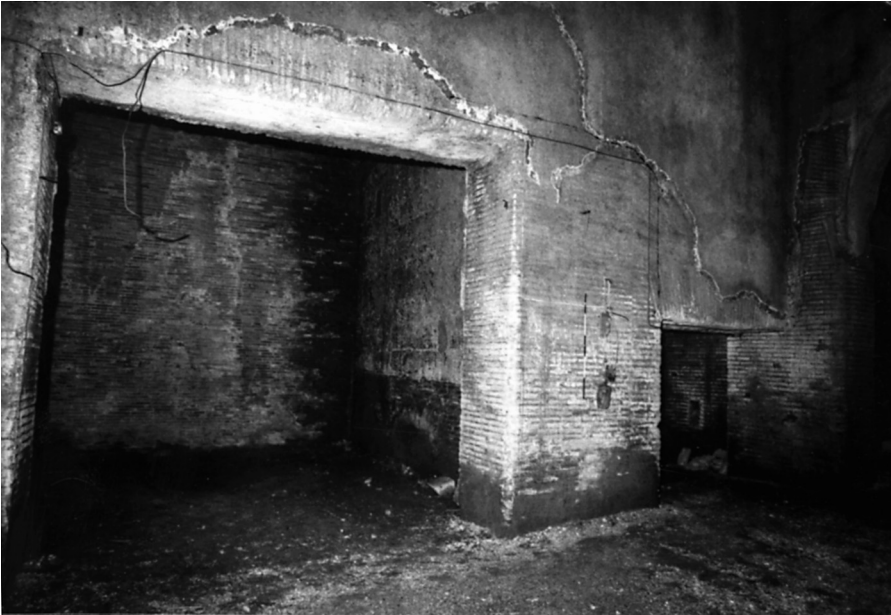
7. Room 39: Overview of the west side. L–R: Type E masonry with large doorway to the West Court; seam between Type E and Type C (to the right of the meter); Type C with small doorway to Corridor 19; doorway, with arched lintel, to Staircase 38.
