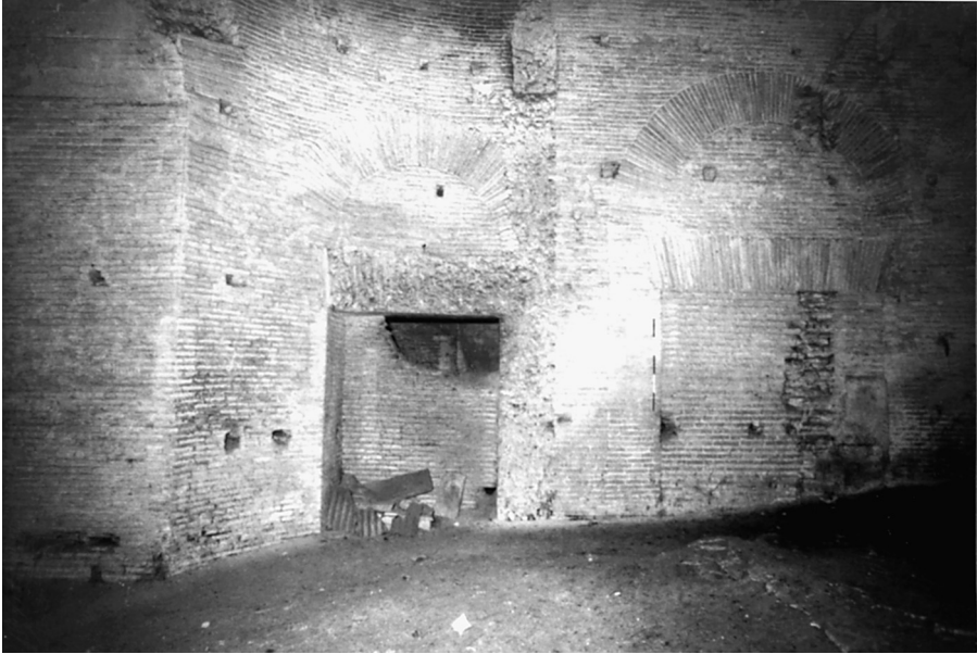
63. Room 51: West side, south half. L-R: alcove in the apse (left edge of photo, Neronian phase 2 Type G); west half of the apse (Type G), with d50.51S (Fig. 62); scar from Neronian phase 1 cross wall forming the right (north) jamb of d50.51S and most of its flat arch lintel; Remnant of the Neronian phase 1 wall to the right (north) of the scar (more clearly visible in Figs. 62 and 65); Neronian phase 2 Type F wall fabric (with meter); fill in d50.51N (Fig. 62), including a prepared semibond scar; more Type F to the right edge of the photo
