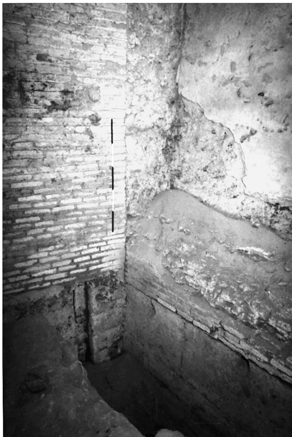
19. Room 54: Detail of the southeast corner, corresponding to Figure 17.5. Bottom left: Unfaced Neronian phase 1 foundation abutting the Type B ashlar foundation. Left: Neronian phase 1 Type E facing abutting imbedded Type B wall fabric. Right (above Type B): Unfaced Type C core concrete, originally cast against the then standing Type B wall.
