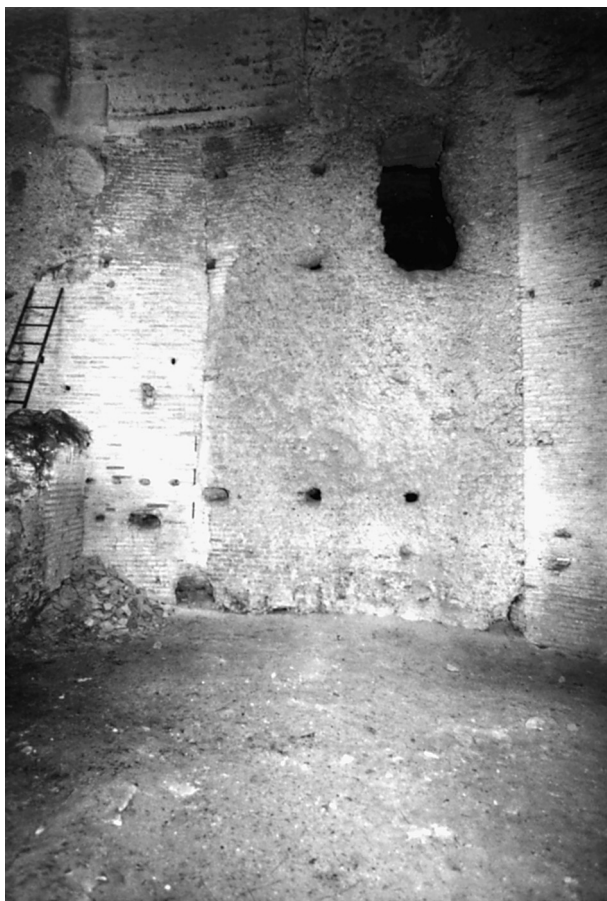
59. Room 51: East side, south half. L-R: Type J cross wall (with ladder above it) abutting the Neronian phase 2 Type G facing; Type G patch itself (meter at the right edge); Type X facing showing from behind the Type G (just right of the meter); wide patch of exposed Type X core concrete (with large hole high up) where Room 66 was trimmed off to make way for Neronian phase 2; Type G facing in the apse (right edge of the photo).
