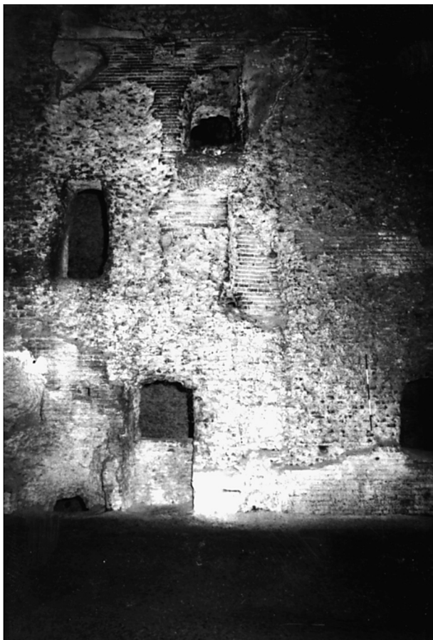
23. Room 36: The north half of the east side. L–R: Post-Neronian door and window cut between Rooms 36 and 37; vertical scar where a bonding Type C wall was razed, at the top of which the Type C material has fallen away, exposing the Type Y facing imbedded in the wall; Type C wall (with its facing retained at the bottom); Window to Room 56 (right edge of the photo).
