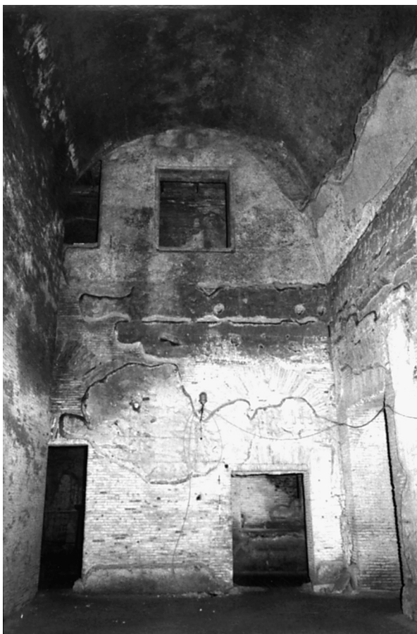
51. Room 44: South half (Room 44B in Fig. 42), overview to the east. L–R: Trajanic Type M foundation wall partially blocking the central doorway to Room 45A. The Othonian Type L wall between Rooms 44 and 45A with decoration remnants and, at the top, the profile of the original Neronian phase 2 vault preserved in the lighter colored decoration (dark Trajanic vaults above); Neronian Type F south side wall with doorway to Room 49.
