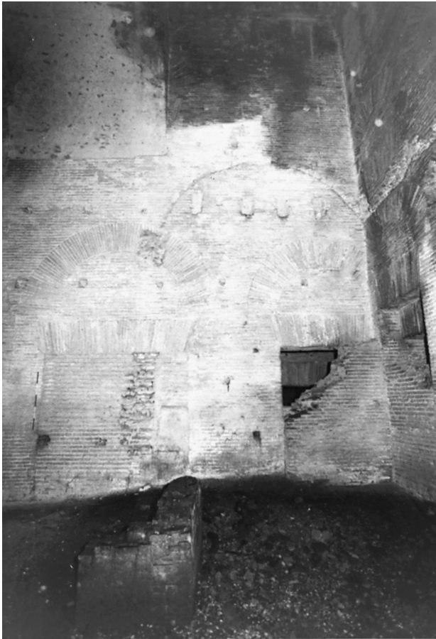
64. Room 51: West side, north half. L-R: Neronian phase 1 masonry (sliver at left edge of photo); Neronian phase 2 Type F masonry, with meter; fill in d50.51N (Fig. 62), with prepared semibond scar; Type F masonry; d45A.51 (Fig. 62); Partially damaged masonry slab set inside Room 51, converting d45A.51 into a niche (when seen from Room 45A); south side of Room 45.
