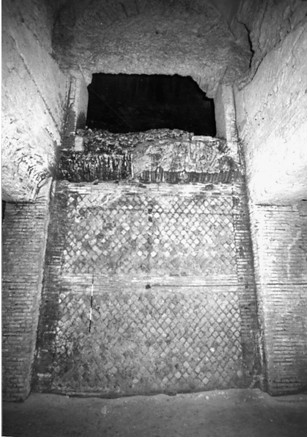
13. Room 67: The southeast end, viewed from inside the room. An example of a large, low window over a doorway (later filled in with opus reticulatum ) where no exterior colonnade was intended, analogous to the original Neronian phase 1 design for the West Court (20), before it was decided to install a colonnade (cf. Figs. 31 and 32).
