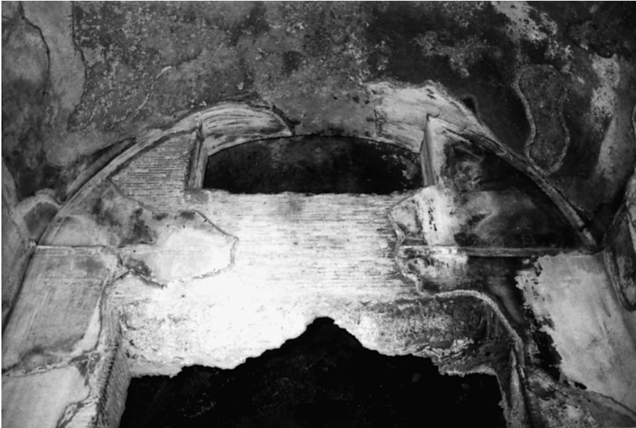
33. Room 27: The north end skylight window, viewed from the interior of the room (from the south). This is entirely of Neronian phase 2 masonry, lacking the seams around the small skylight that the original larger windows of Neronian phase 1 left around the rest of the north skylights in the West Suite.
