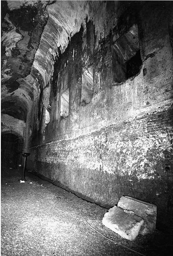
25. Corridor 92: The south side of the west end, looking southeast. The wall is Type C (or earlier) and the windows are the skylights cut through it when Rooms 93–101 were added to the south of it in Neronian phase 2. The ramp for the water cascade in Room 102 appears in the distance at the left.
