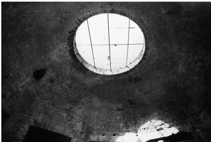
78. Room 128: Overview of the dome (looking to the west).
