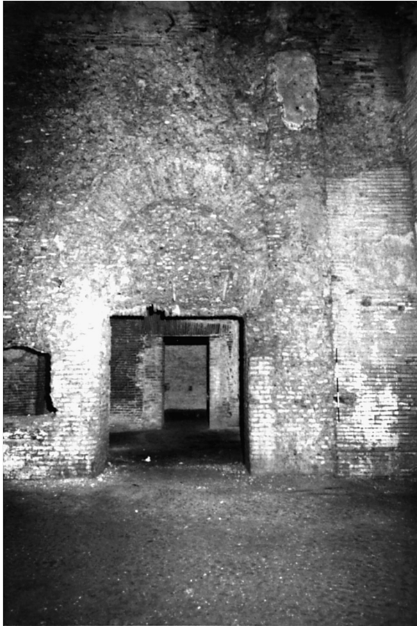
24. Room 36: The south half of the east side. L–R: Window to Room 56 (left edge of photo); Type C masonry surrounding the doorway to Room 56, including the lighter facing forming the south (right) jamb; vertical scar where a bonding Type C wall was razed; seam between Type C (pre-Neronian) and the Neronian phase 1 Type E added to the south (right) of it, continuing to the far right edge of the photo. The meter is on the Type E next to this seam.
