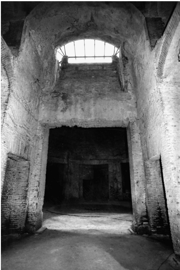
75. Room 123: Overview to the southeast, including a view out of the vault haunch clerestory.
