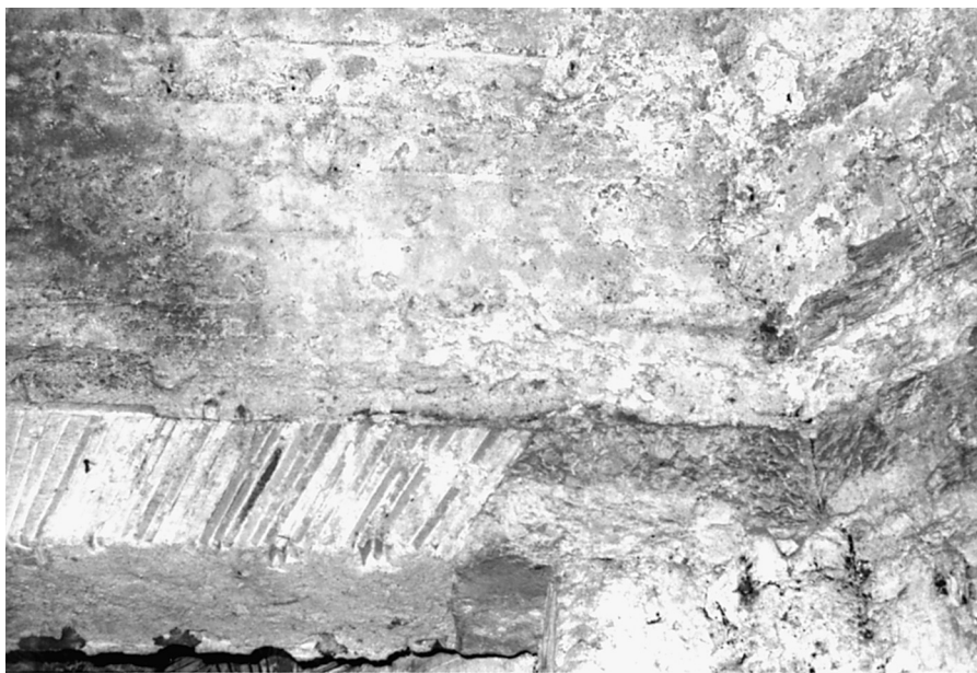
79. Room 128: Detail above the southeast lintel, including formwork impressions and remnants from the setting bed for the dome mosaics.
