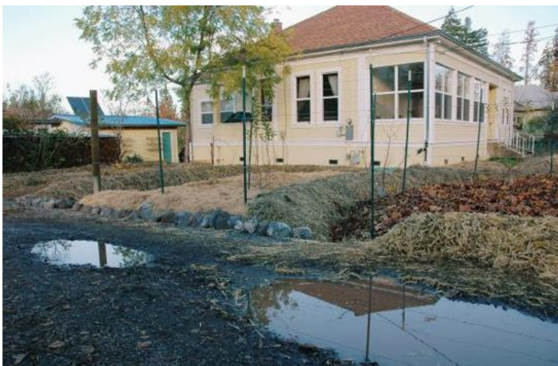
Newly installed earthworks including swales, berms, permeable pathways, French drains, and keyhole planting in this Willits, California yard. The standing water seen in the foreground was common throughout the site before the earthworks, compost, and mulch were installed. Posts for trellising the mini-food forest can be seen where the lawn once was. In the background is the downspout leading to the water storage under the house and to the left the garage/guest room features trellises for vertical gardens in front of it. Design by Maximillian Meyers of the Mendocino Ecological Learning Center. PHOTO BY MAXIMILLIAN MEYERS.
