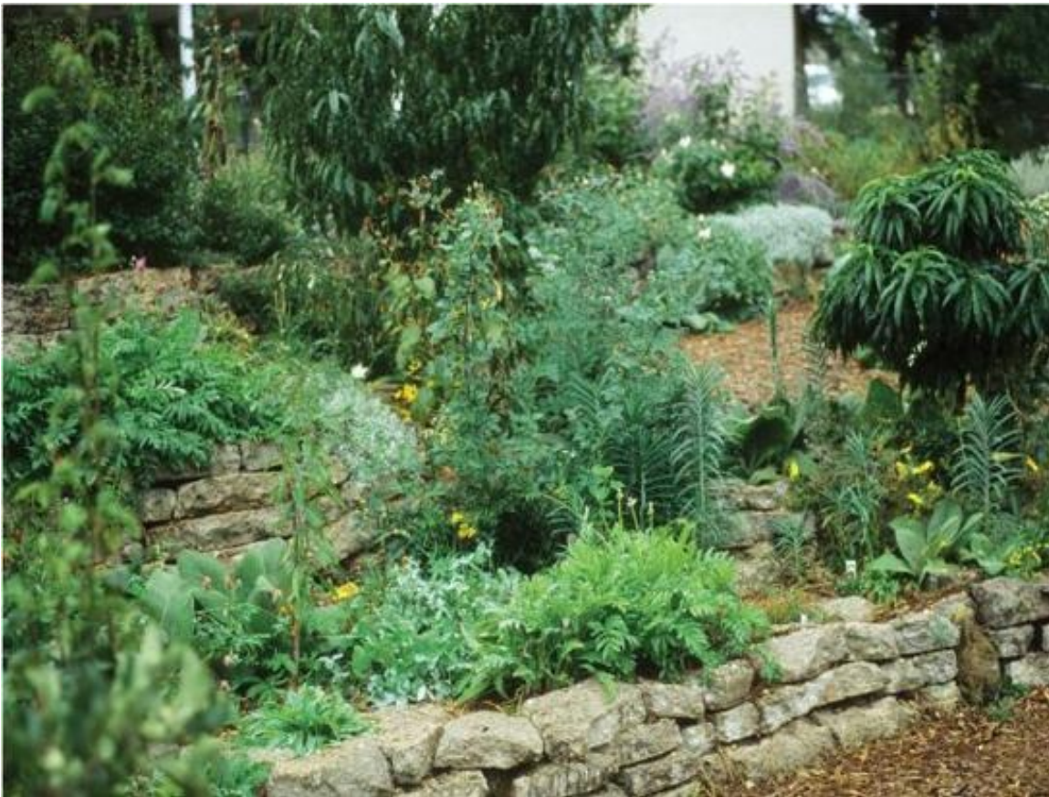
Terraces made from broken concrete (“urbanite”) hold perennial food and habitat plants in the Los Alamos, New Mexico garden of Mary Zemach, designed by Ben Haggard and Nate Downey, Santa Fe.
