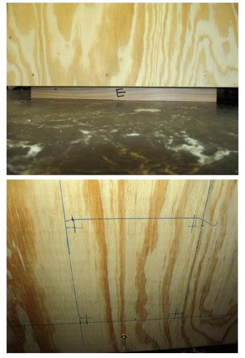
Drill  $\frac{3}{16}$  holes for the mounting bolts for the fan, and then use a reciprocating saw to cut out a hole for the air to blow through.
