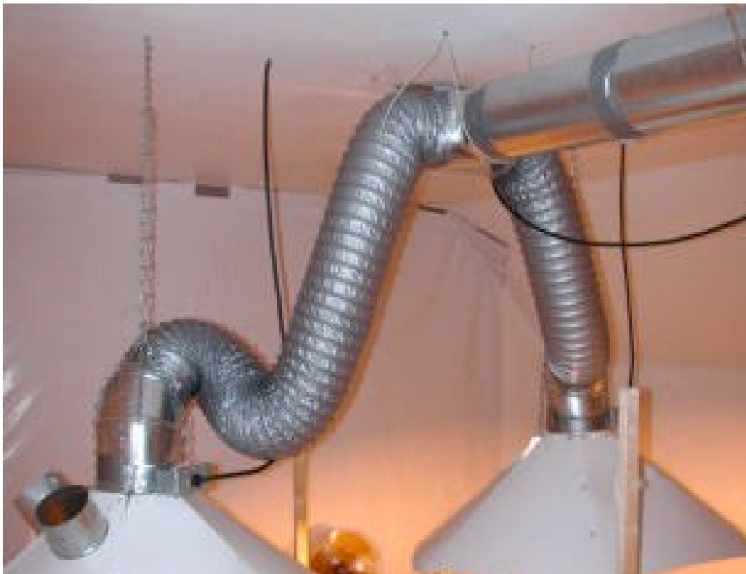
Figure 5.12 - This picture shows two air-cooled hoods attached to their respective air ducts. This photograph is by Chimera.
