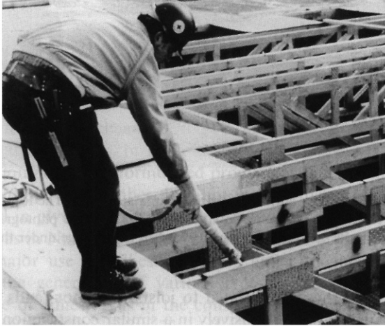
FIGURE 1.5 A construction worker applies a mastic adhesive to the joists in a home construction project. The use of a mastic adhesive in such an application provides for a quieter floor
