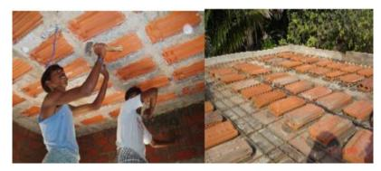
FIGURE 20.3 Reinforced cement concrete filler slab.
