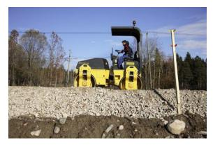
FIGURE 17.1 Road building using reclaimed concrete.
