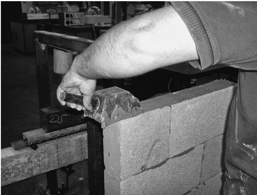
Figure 13.4 Application of thin layer mortar
