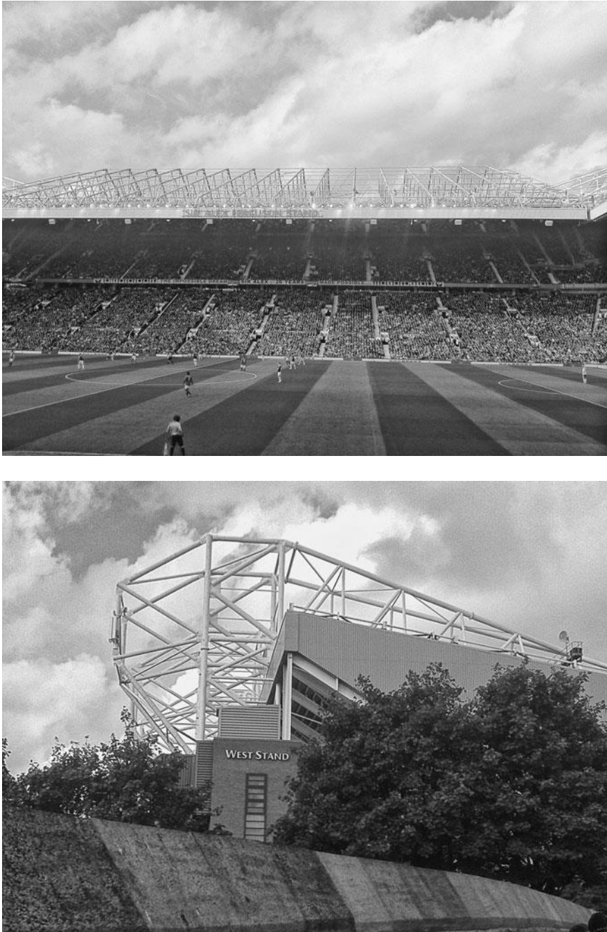
Figure 8.4 Old Trafford Stadium, home to Manchester United Football Club, and the cantilever roof structure, which is made from steel ( www.manutd.com )
