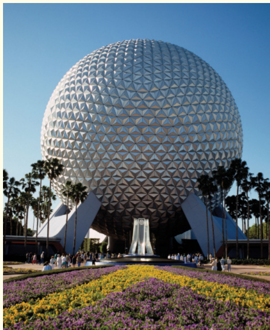
An example of a geodesic dome (of the type whose design was pioneered by Buckminster Fuller) forms part of the entrance to EPCOT Center, Disney World, Florida. It is 180 feet high with a diameter of 165 feet.
