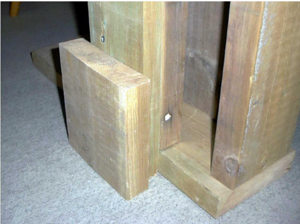
Proposed Whisker, additional sideways support. Fixed to give good support to floor or table, by way of at least 5 screws. This should really make these stands strong as cast-iron supports!
