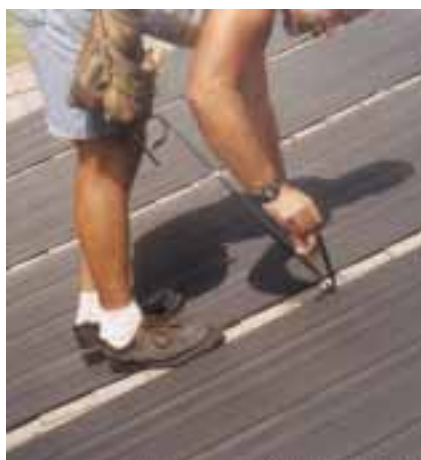
Collector risers are held in place during strong winds by rubber-coated stainless steel straps. The straps are threaded through stainless steel butterfly clips that are screwed to the roof.
