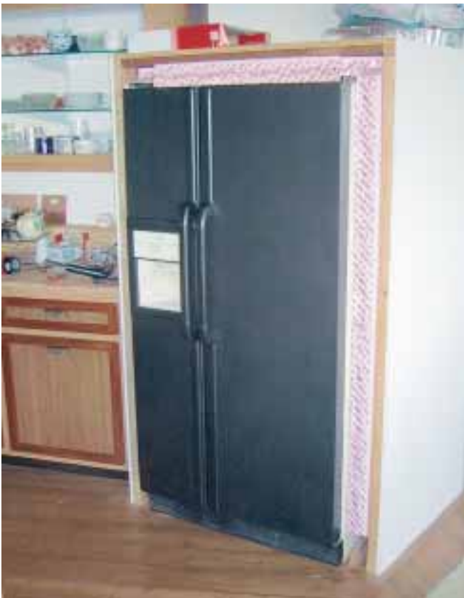
Refrigerator in enclosure, lined with foam insulation.
