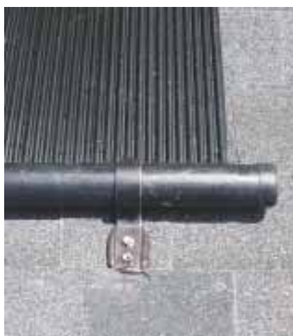
Metal pipe clamps \frac{1}{2} inch larger than the pipe hold PVC pipe and collector headers securely to the roof. A generous amount of quality sealant is used to prevent roof leaks.
