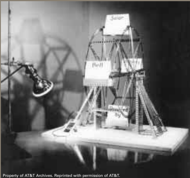
One of Bell's first silicon solar modules powers a Ferris wheel built from an Erector set at the first public demonstration on April 25, 1954.
