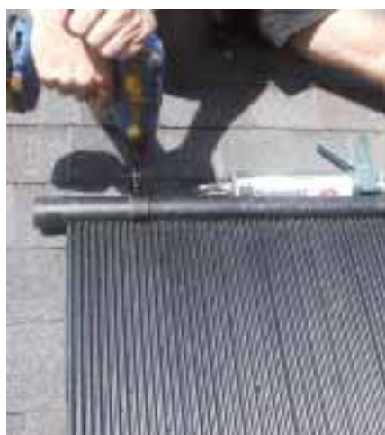
Metal pipe clamps \frac{1}{2} inch larger than the pipe hold PVC pipe and collector headers securely to the roof. A generous amount of quality sealant is used to prevent roof leaks.
