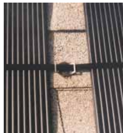
Collector risers are held in place during strong winds by rubber-coated stainless steel straps. The straps are threaded through stainless steel butterfly clips that are screwed to the roof.
