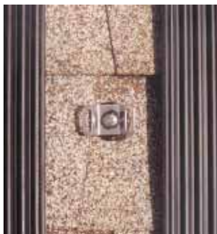
Collector risers are held in place during strong winds by rubber-coated stainless steel straps. The straps are threaded through stainless steel butterfly clips that are screwed to the roof.
