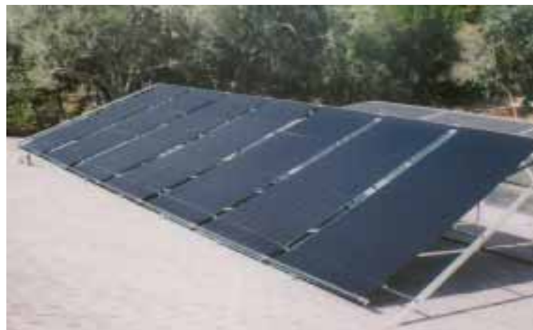
South-facing solar collectors on a north-facing roof.
