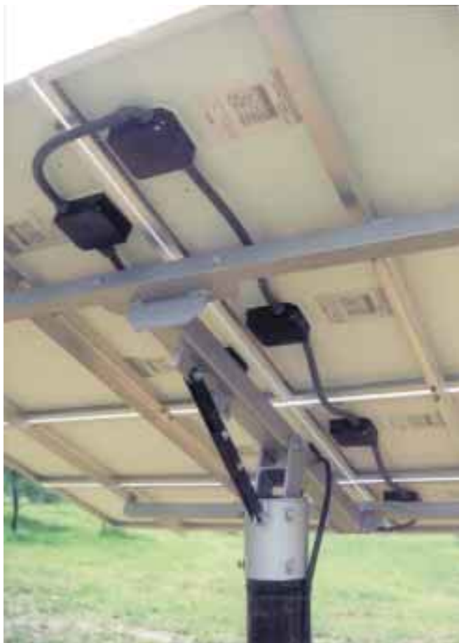
The twenty-four Direct Power and Water PV racks can be adjusted for seasonal angle in less than one minute each.
