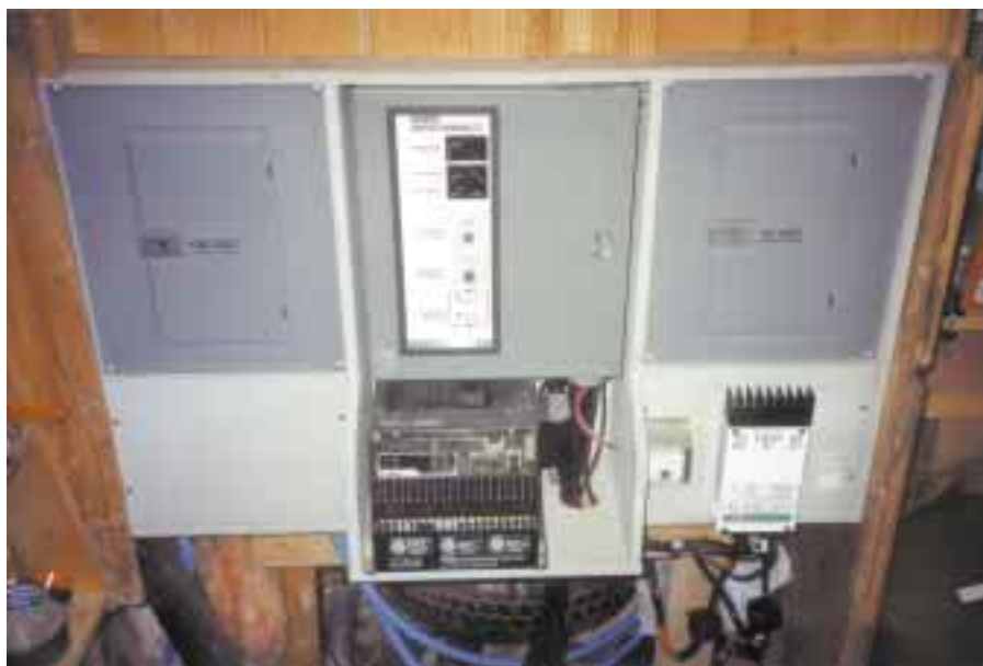
The power panel includes a modified sine-wave inverter and 60 amp controller.
