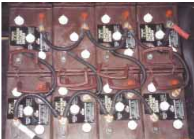
Eight Trojan L16Hs store 1,580 amp-hours at 12 volts.
