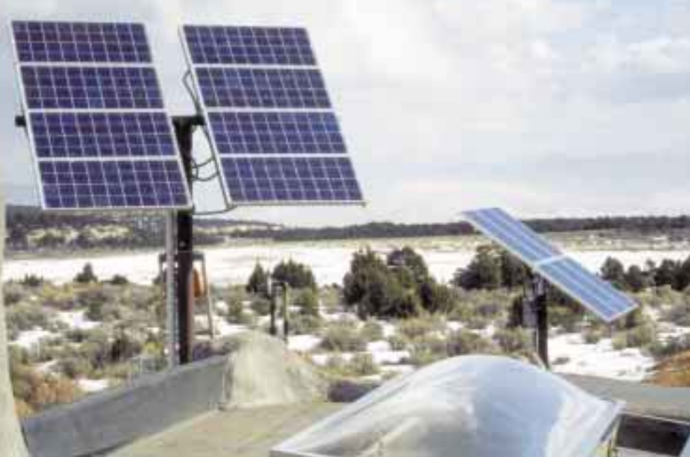
888 watts of PV, and a small wind generator cover the electrical loads.
