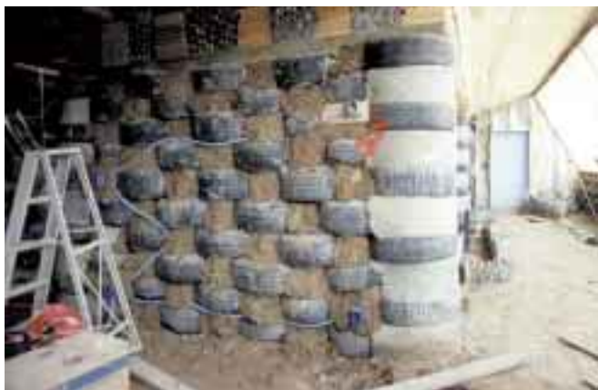
Recycled tires with rammed earth fill make cheap and energy efficient walls.
