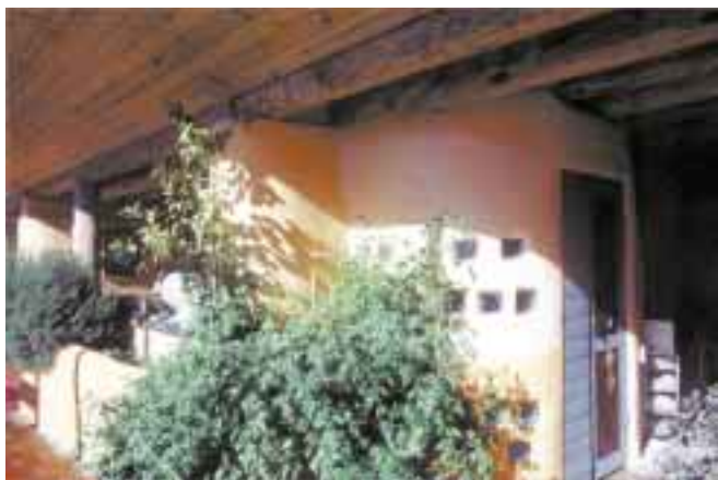
Earthen stucco creates energy-storing thermal mass.
