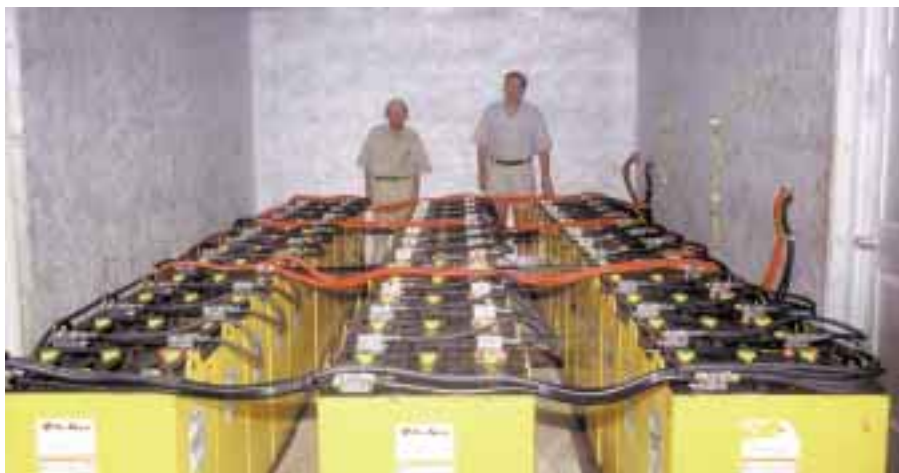
Eighteen tons of Deka lead-acid batteries provide 11,223 amp-hours of storage.
