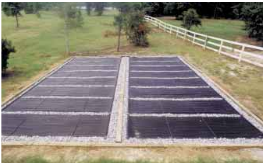
Efficiency, load shedding, and solar like this pool heater, were all important for the PV system to meet the projected loads.
