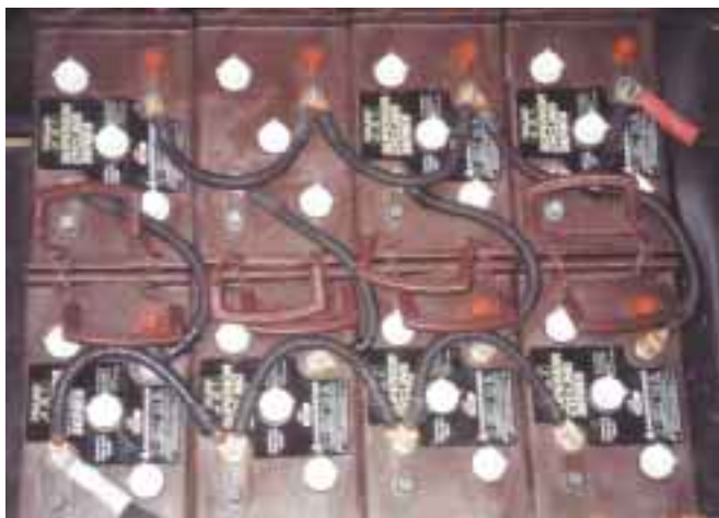
Eight Trojan L16Hs store 1,580 amp-hours at 12 volts.
