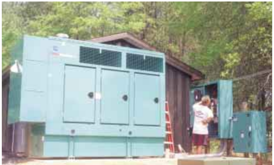
A huge 100 kilowatt Onan Cummins diesel generator provides backup.
