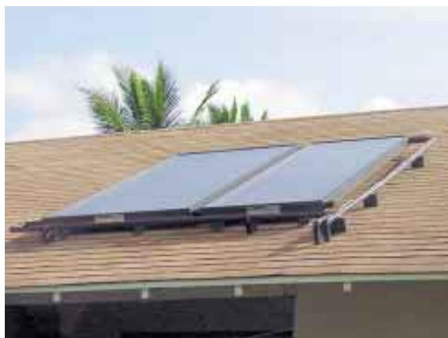
Two roof-mounted flat plate collectors.
