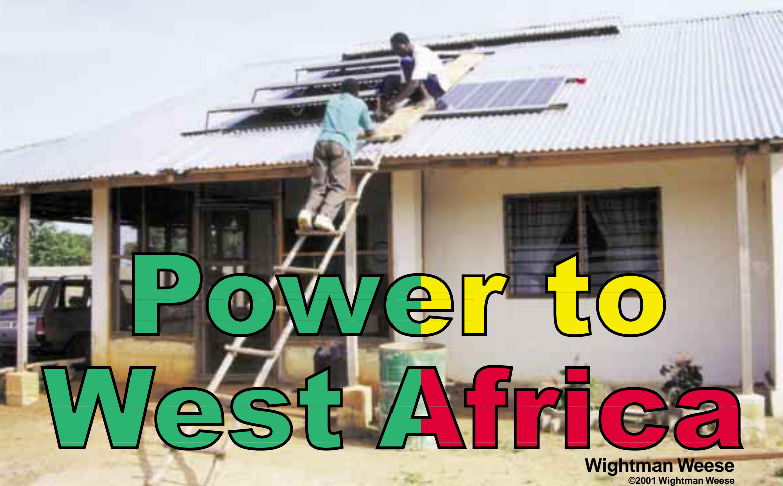
The crew installing the fourth array. The photovoltaics were set at 15° south.
