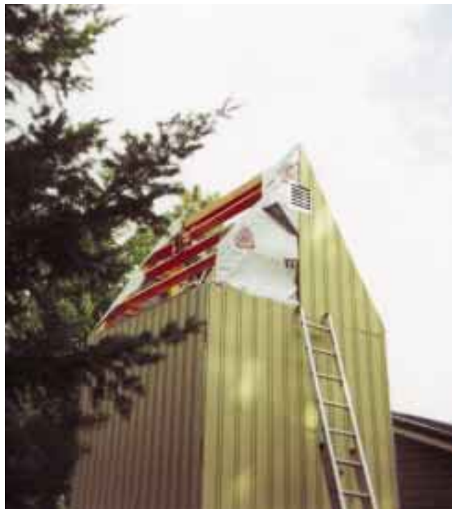
Norma finishes up the Power Tower's siding, which was recycled from a storm damaged barn.
