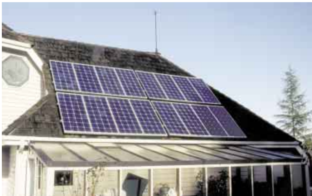
Sixteen AstroPower PV modules, for a total of 1,920 rated watts, are mounted on the south-facing roof above the greenhouse.
