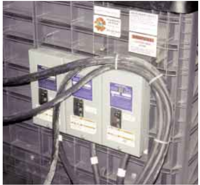
Generator, utility power, and main output breakers.
