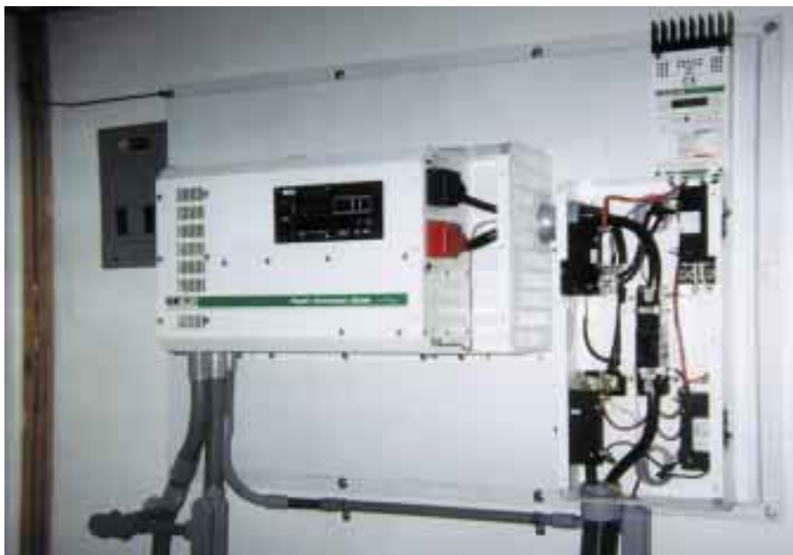
Trace SW2512 inverter, DC250 disconnect box, and C60 controller in the Power Tower's first floor room.
