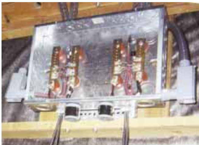
The custom PV combiner box was made from an electrician's leftover bits and pieces.
