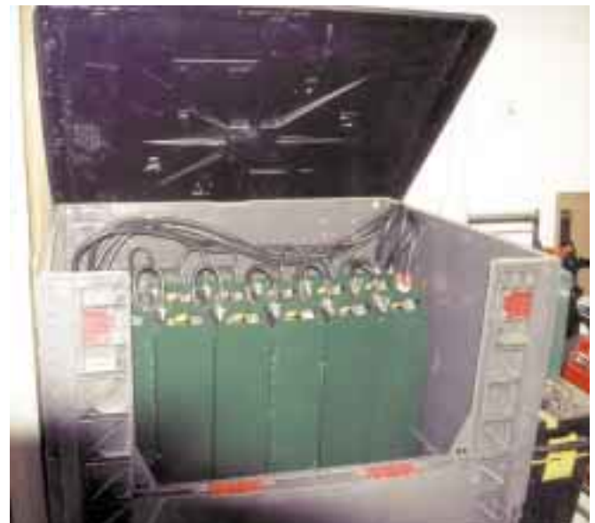
The battery module provides vented containment for the twelve IBE lead-acid cells.
