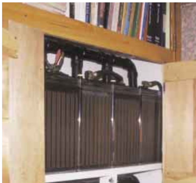
The Barkers challenged conventional battery assumptions—the twenty-year-old, reclaimed bank of flooded lead-acid cells proved worthy.
