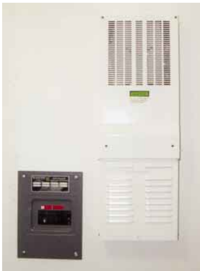
The utility-intertie Trace Sun Tie 2500 sine wave inverter (right) and the upstairs AC subpanel.
