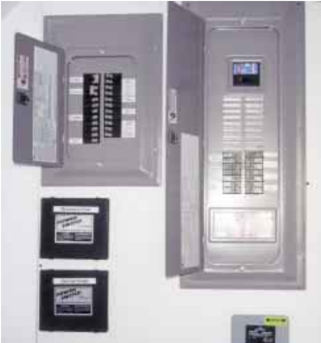
The main grid panel and subpanel with the automatic transfer switches for the ovens, below.
