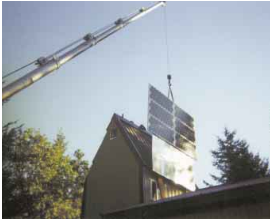
A crane made it easy to install the wired and racked PVs. The rack space covered with sheetmetal is where four more modules will be installed later.
