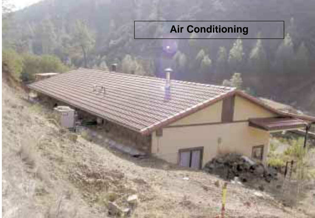
The Servel three-ton gas-fired cooling unit behind the house.
