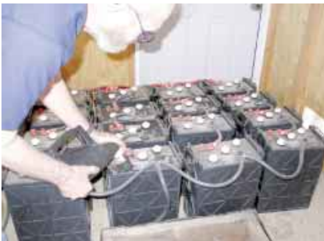
Sixteen Trojan L-16s make up the new battery bank.
