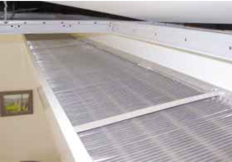
Looking down from the ceiling—the cooling fins create surface area for maximum air contact.
