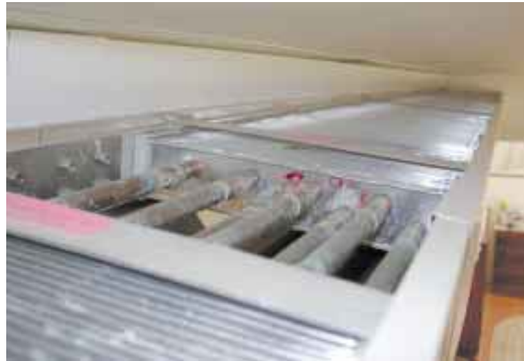
Nine finned copper pipes carry cool water through the heat exchanger.
