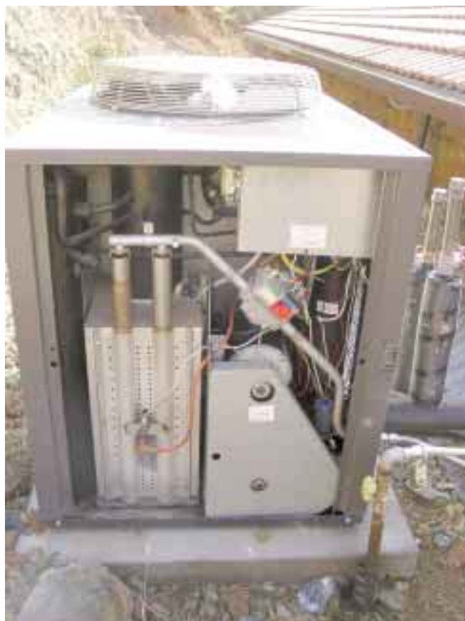
Inside the Servel air-cooled absorption water chiller.
