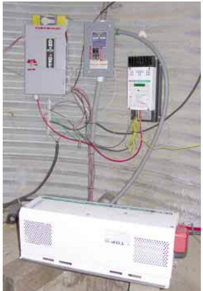
The Trace DR3624, C-40, fuses, and disconnects.
