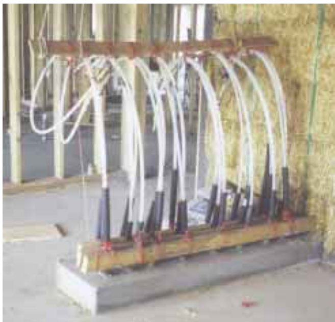
Tubes gathered and ready for a manifold.
