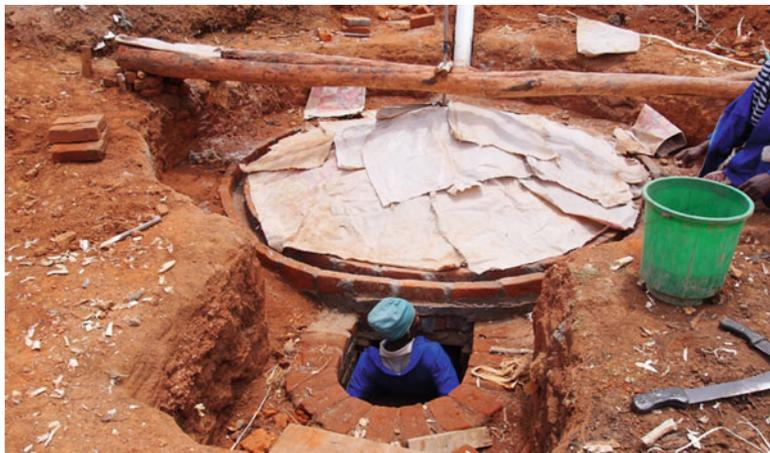
**Fig. 5.15** A below-ground biogas digester being constructed in Malawi (courtesy P. Dauenhauer)
