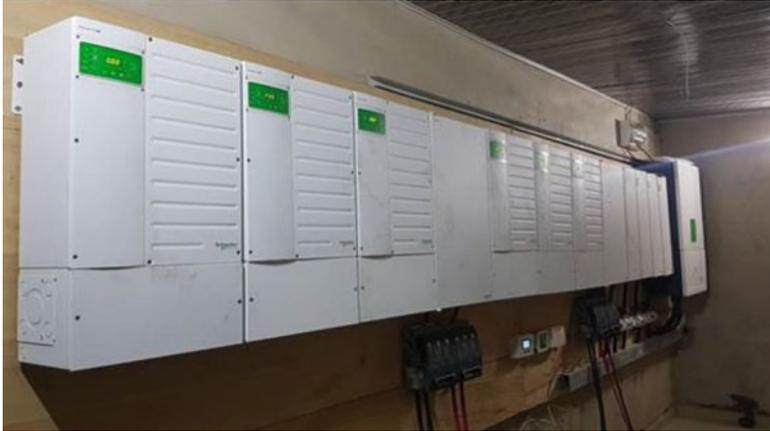
**Fig. 9.3** The control room of a large mini-grid in Nigeria, consisting of inverters, charge controllers, and system monitoring equipment (courtesy of GVE Projects)
