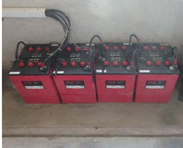
six series-connected lead–acid cells. Only two electrodes are accessible. They are known as the “terminals” of a battery. One is positive and the other negative, just like an individual cell. The load or charging circuit is connected to the terminals. Several batteries can be connected together to form a battery bank as in Fig. 8.4. Series connections increase the overall voltage; parallel connections increase the available current.
