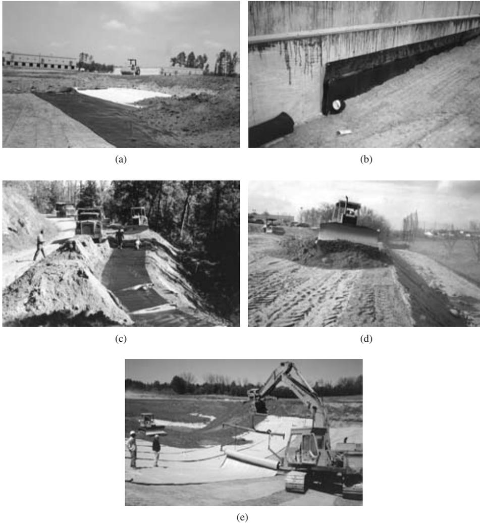
**FIGURE 4-21** Examples of use of geosynthetics (Courtesy of C.F.P. Inc.). (a) Geotextile stabilization, (b) Geocomposite drainage panel, (c) High-strength geotextile (slide repair), (d) Geogrid reinforced steepened slope, and (e) Geosynthetic clay liner.
