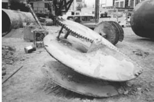
**FIGURE 11-6** Steel casing used in drilled shaft construction.
