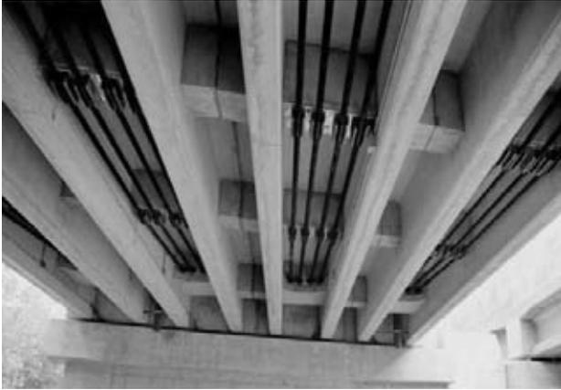
**FIGURE 11.9** Strengthening a concrete bridge with FRP bars.
