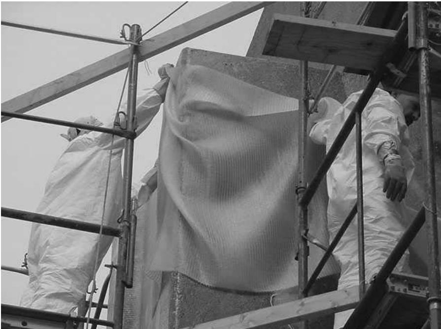
**FIGURE 11.6** Wrapping an old structure with glass fiber-reinforced polymer (FRP) composite (Wabash Avenue pier, Baltimore, MD).
