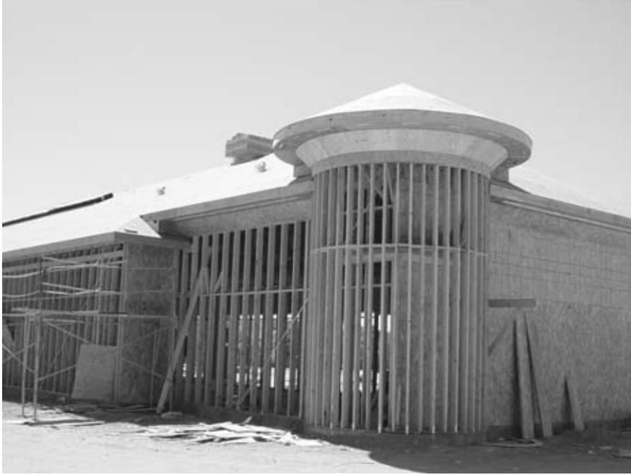
FIGURE 10.1 Wood frame used for building structural support.
