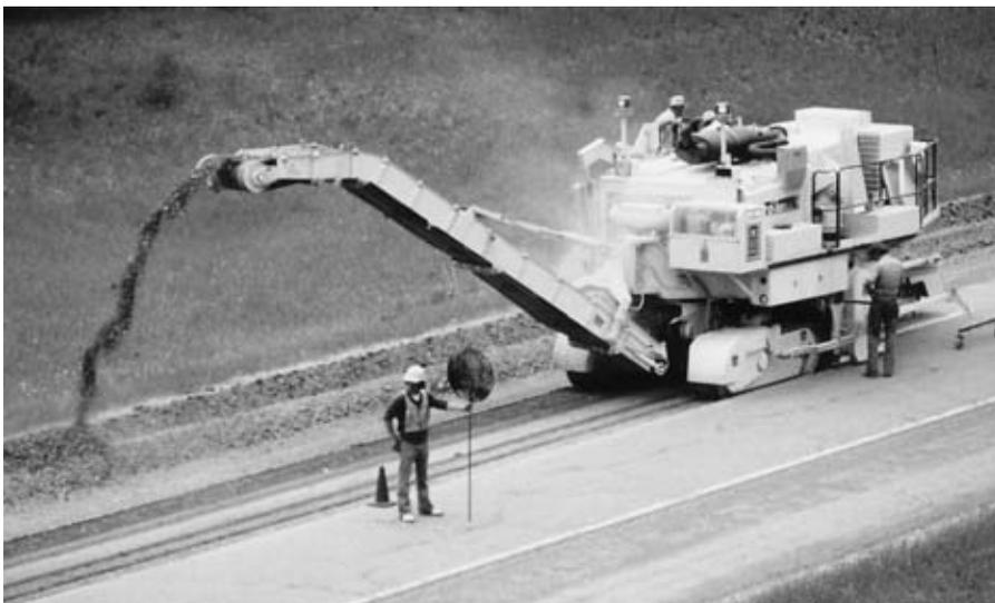
FIGURE 9.39 Milling old pavement.
