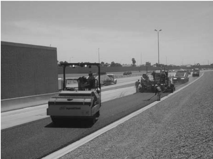
**FIGURE 9.4** Compaction of hot mix asphalt.
