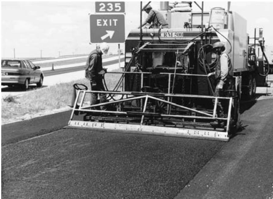
**FIGURE 9.6** Applying microsurfacing for preserving existing pavement.
