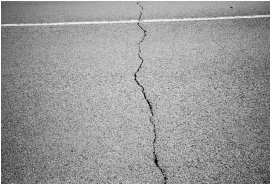
**FIGURE 9.8** Thermal cracking resulting from the use of too stiff asphalt in a cold climate area.
