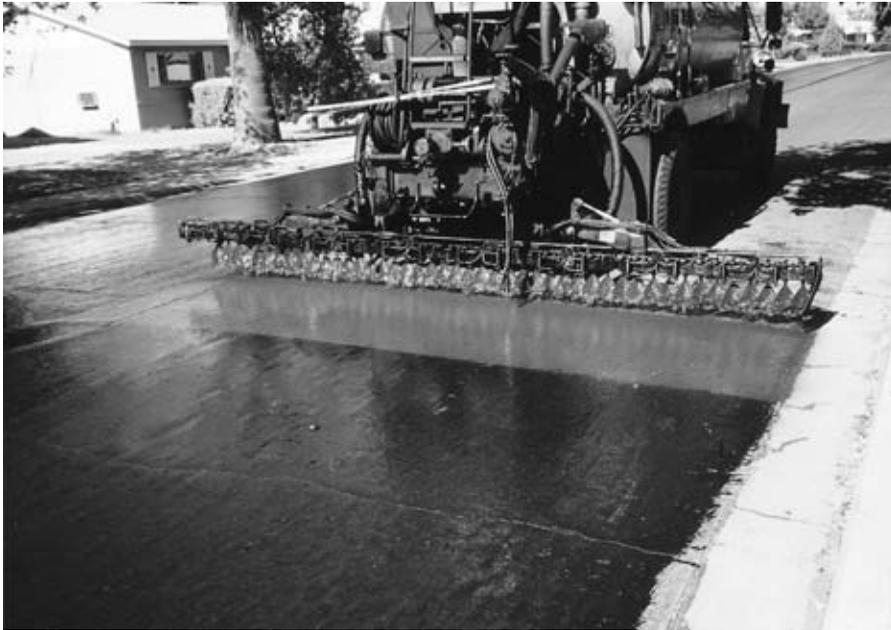
**FIGURE 9.5** Applying fog seal for preserving existing pavement.
