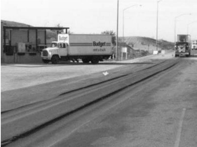
**FIGURE 9.9** Rutting that could result from the use of too soft asphalt.
