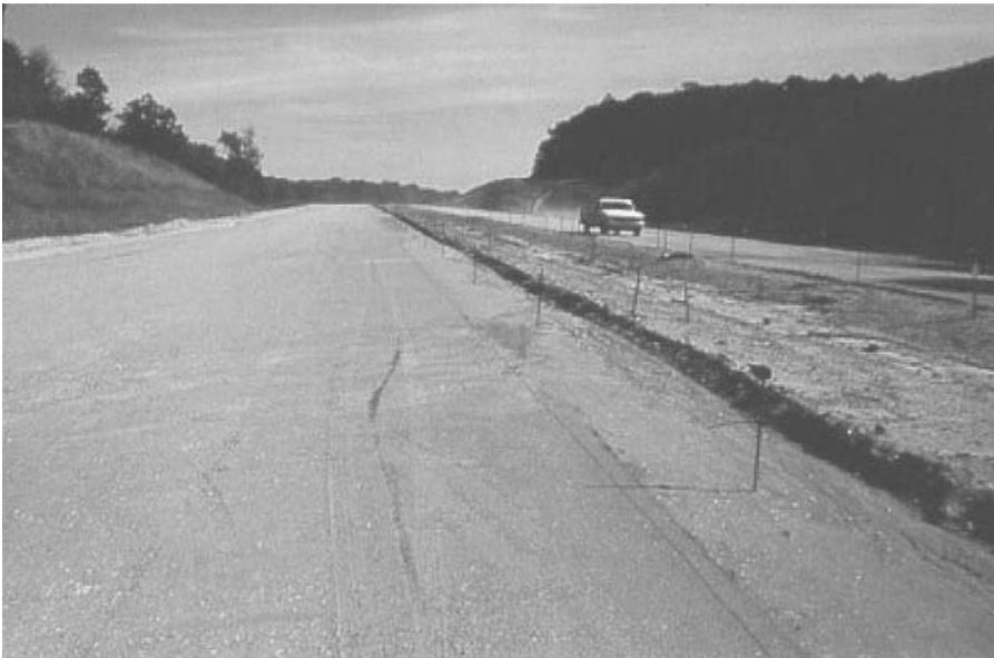
**FIGURE 5.2** Compacted aggregate base before placing the hot-mix asphalt or portland cement concrete layer of a paved road.
