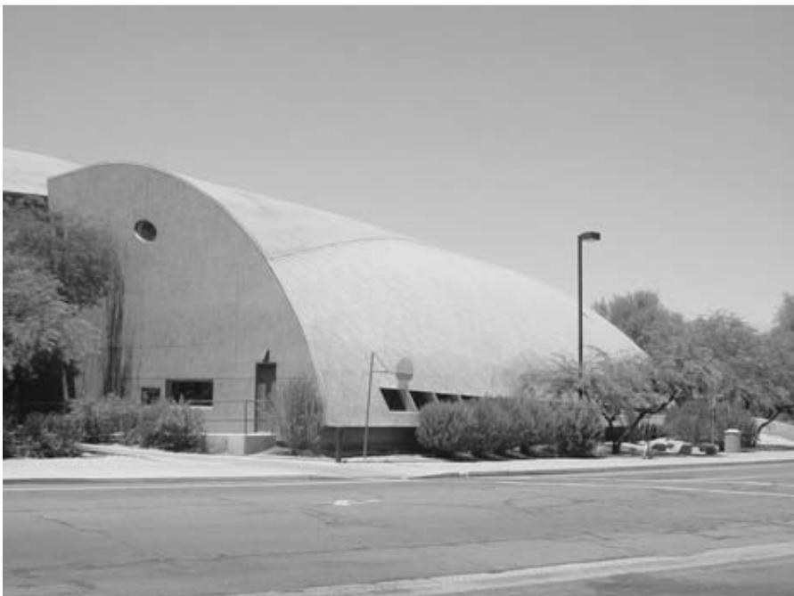
**FIGURE 4.2** Building facade made of aluminum.
