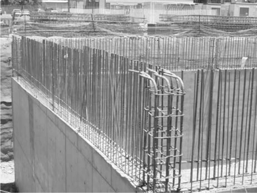
**FIGURE 3.2** Steel rebar used to reinforce portland cement concrete wall.
