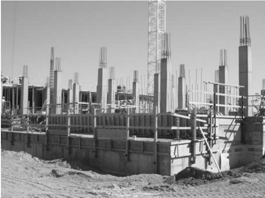
**FIGURE 3.10** Steel rebar used to reinforce PCC columns.
