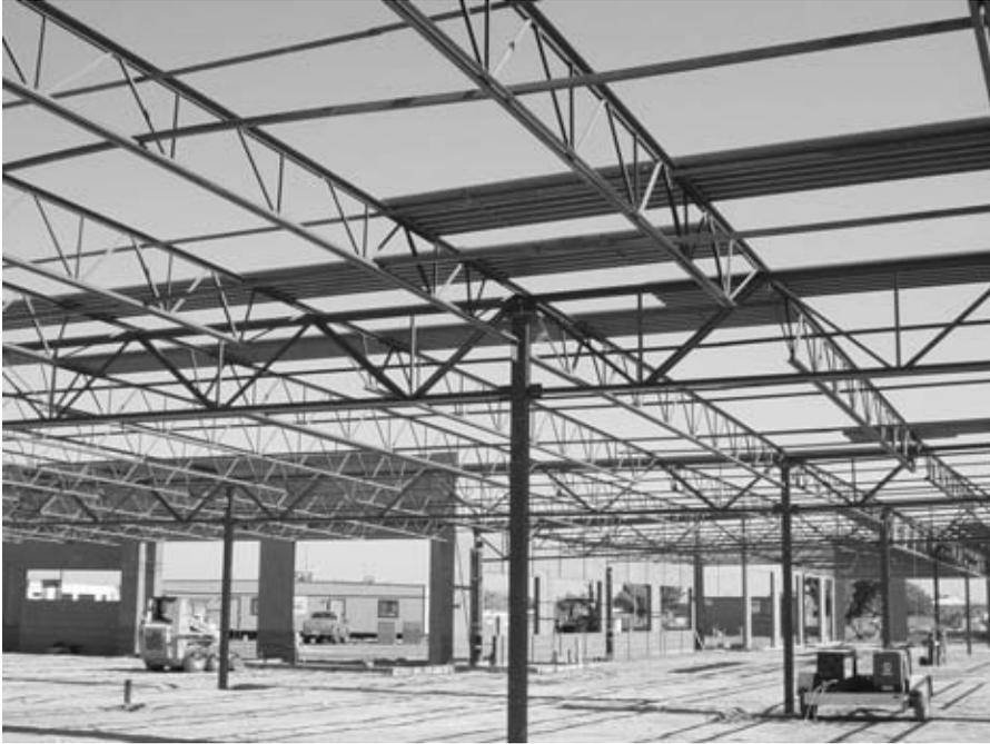
**FIGURE 3.1** Truss made of structural steel for the structural support of a building.
