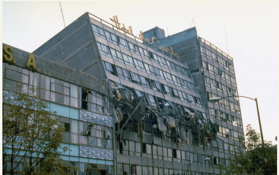
**FIGURE 11.B** During the 1985 Mexican earthquake, multistory buildings swayed back and forth as much as 1 meter. Many, including the hotel shown here, collapsed or were seriously damaged. (Photo by James L. Beck)
