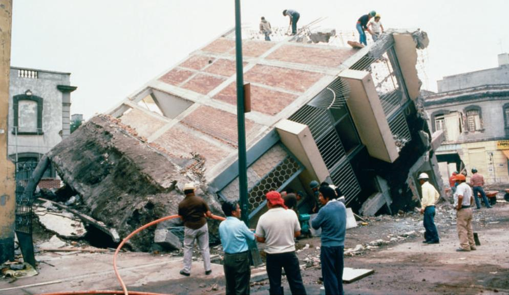
**FIGURE 11.18** Effects of liquefaction. This tilted building rests on unconsolidated sediment that behaved like quicksand during the 1985 Mexican earthquake. (Photo by James L. Beck)
