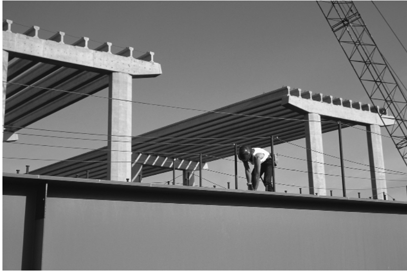
Bridge construction. (PhotoDisc, Inc./Getty Images.)
