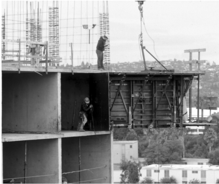
The room tunnel forming system. (Courtesy of Symons Corporation.)
