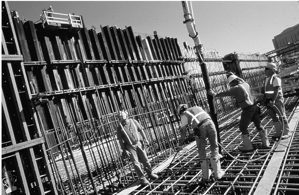
Placing concrete, Big Dig, Boston, MA. (Steve Dunwell/The Image Bank.)
