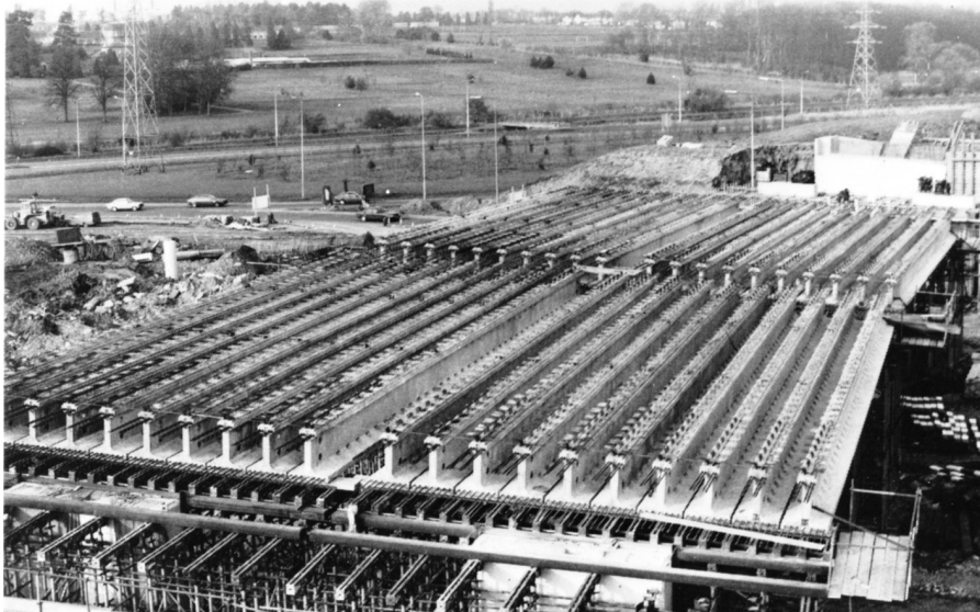
Barnes Meadow Interchange, Northampton, England. (Courtesy of Cement and Concrete Association.)
