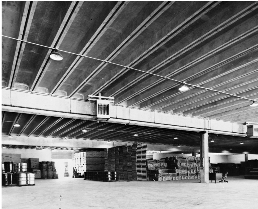
Prestressed concrete channels, John A. Denies Son Company Warehouse #4, Memphis, Tennessee. (Courtesy of Master Builders.)
