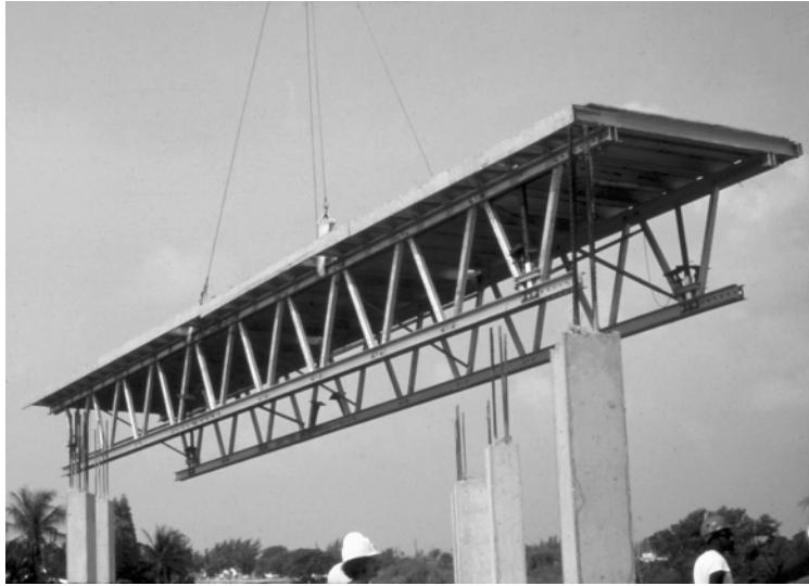
The truss table system for deck forming. (Courtesy of Symons Corporation.)
