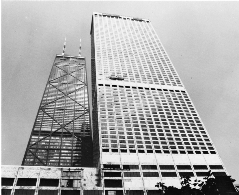
Water Tower Place, Chicago, Illinois, tallest reinforced concrete building in the United States (74 stories, 859 ft). (Courtesy of Symons Corporation.)
