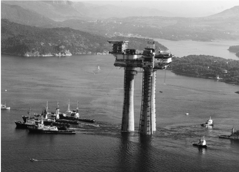
Two reinforced concrete hollow cylinders each 65 ft in diameter and 185 ft high being towed to North Sea location as part of oil drilling platform. (Courtesy of United Nations, J. Moss.)
