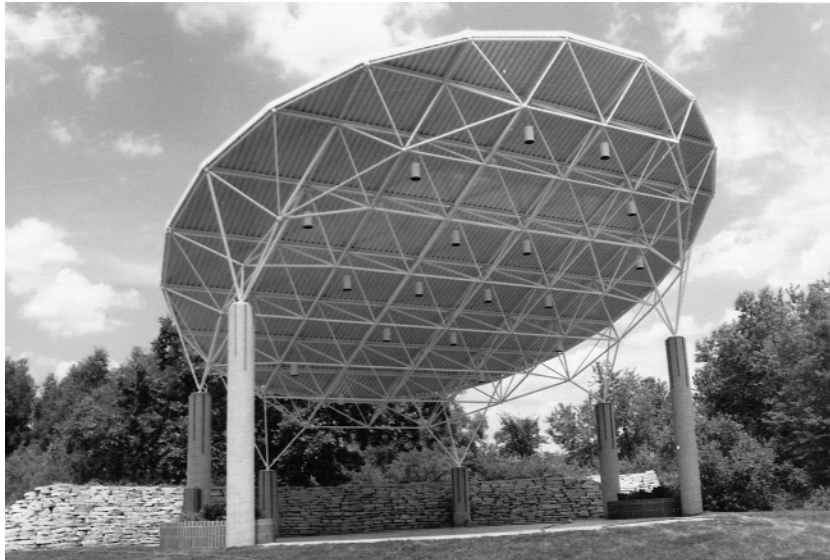
Reinforced concrete bandshell in Portage, Michigan. (Courtesy of Veneklasen Concrete Construction Co.)
