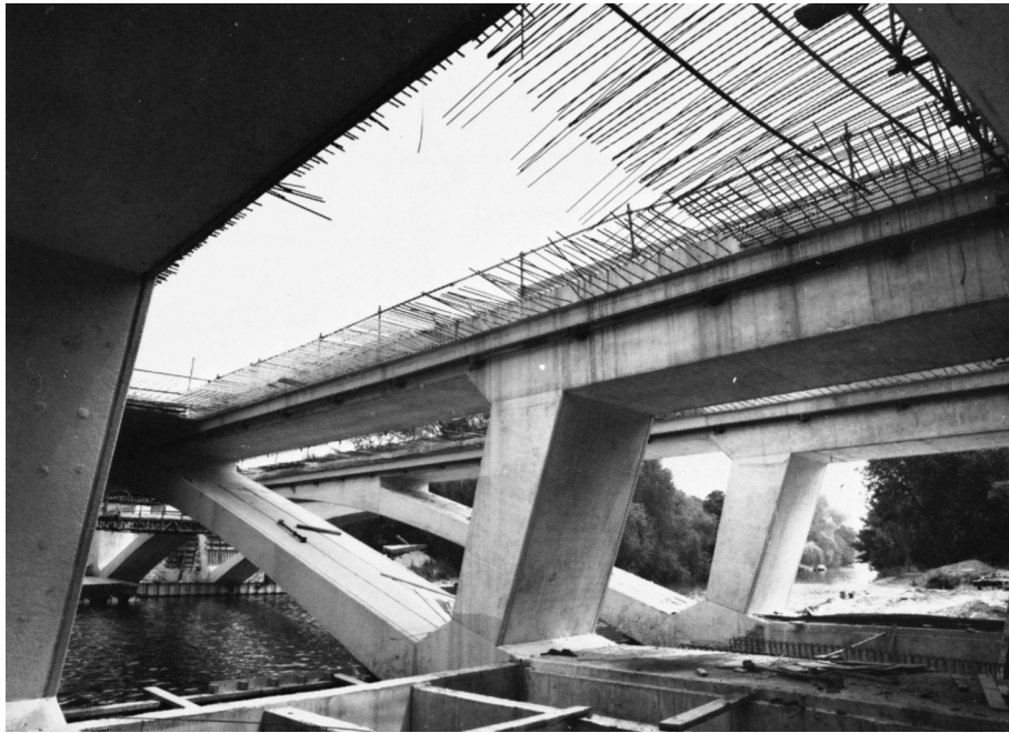
Prestressed concrete Runnymede Bridge over Thames River near Egham, Surrey, England. (Courtesy of Cement and Concrete Association.)
