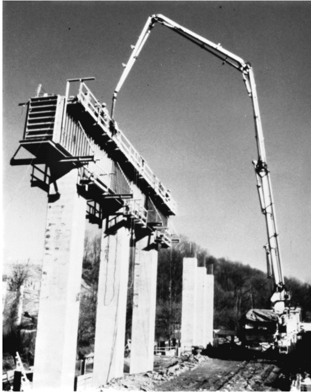
Pennsylvania Southern Expressway, Philadelphia, Pennsylvania. (Courtesy of Economy Forms Corporation.)
