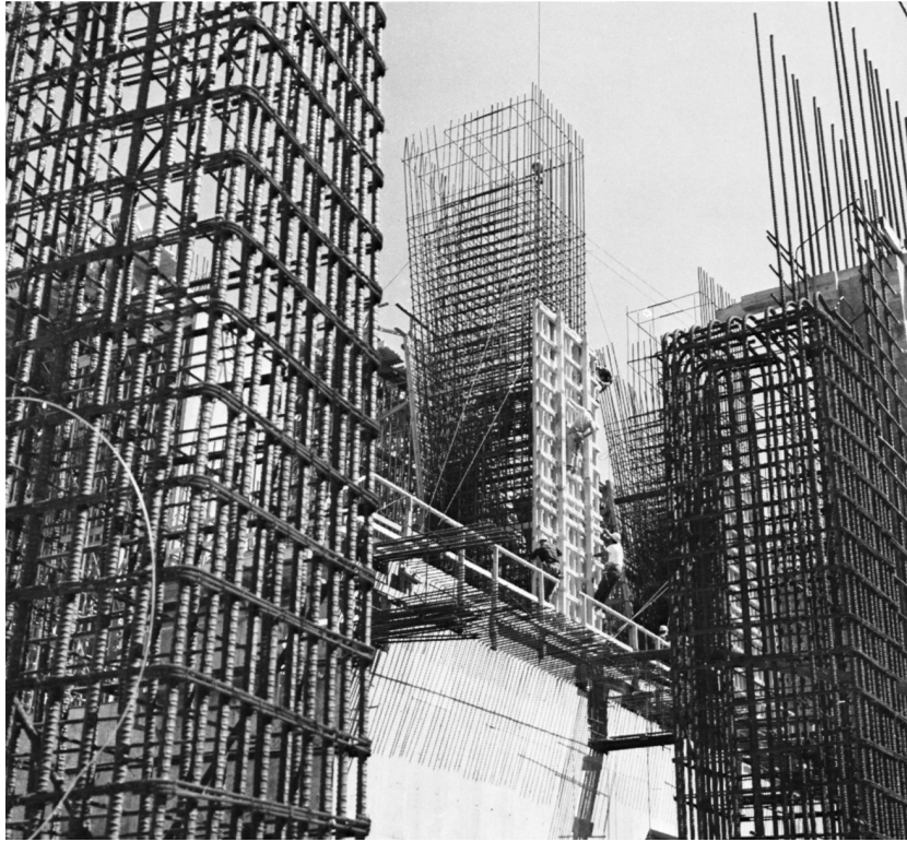
Massive reinforced concrete columns. (Courtesy of Bethlehem Steel Corporation.)
