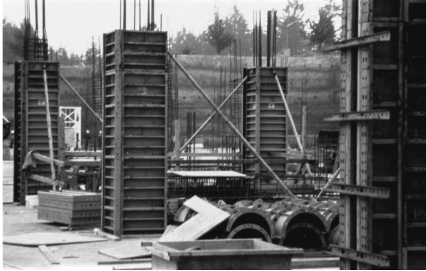
Column forms. (Courtesy of Economy Forms Corporation.)
