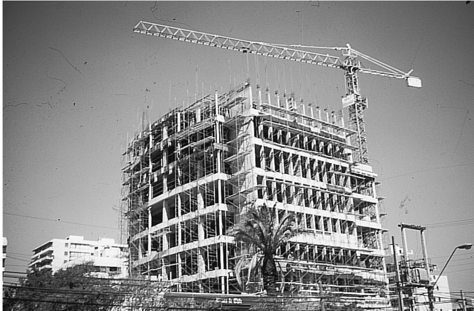
The 16-story Apoquindo Tower, Santiago, Chile. (Courtesy of Economy Forms Corporation.)
