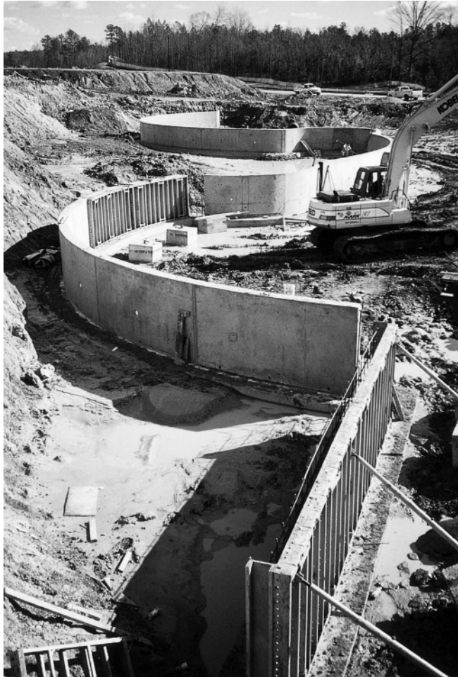
South point water facility, Durham, N.C. (Courtesy of EFCO.)
