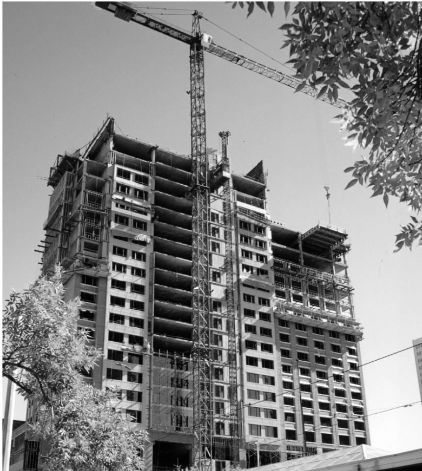
Reinforced concrete building in Calgary, Canada. (Courtesy of EFCO.)
