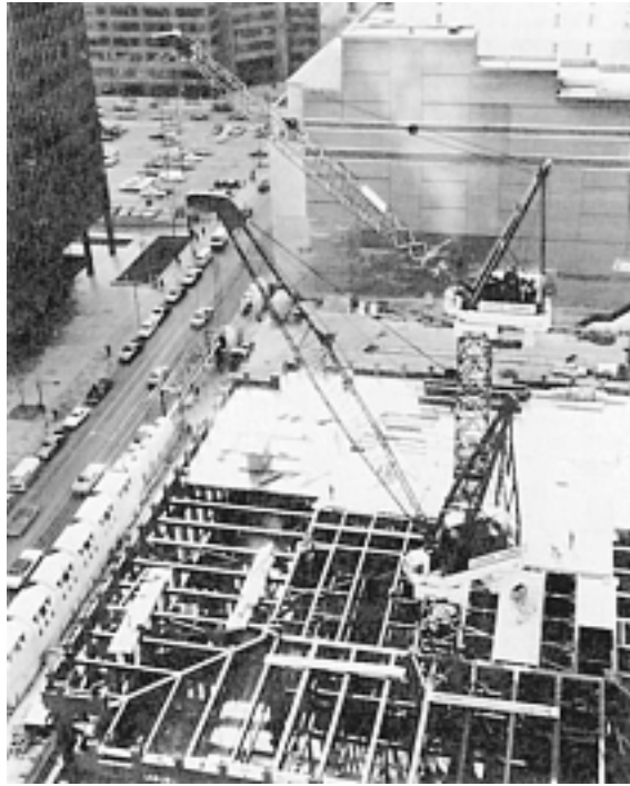
Figure 15–8 Tower crane erecting steel. (Courtesy of FMC Corporation)
