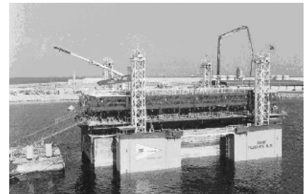
Caisson Construction Valencia, Spain.
