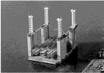
Construction of floating caissons utilized PROSIDYC as a tool to increase production.
