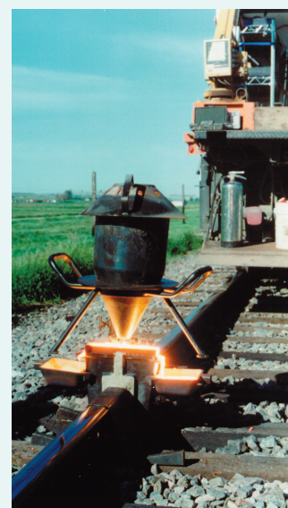
FIG. 3.5 The thermite reaction. Pictured here is a device for making white-hot iron by the reaction of aluminum with iron oxide and letting the molten iron run down into a mold between the ends of two steel railroad rails. The rails are thereby welded together. (Courtesy Orgo-Thermit.)
