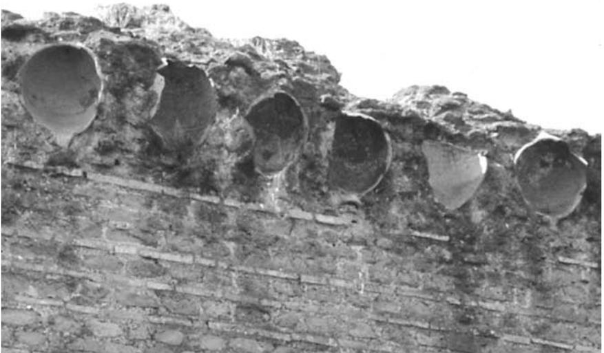
FIGURE 6.18. Dressel 23 *amphorae* reused as lightning elements in *cavea* of Circus of Maxentius, near Rome. Left: general view. Right: detail. Photos: JTP.
