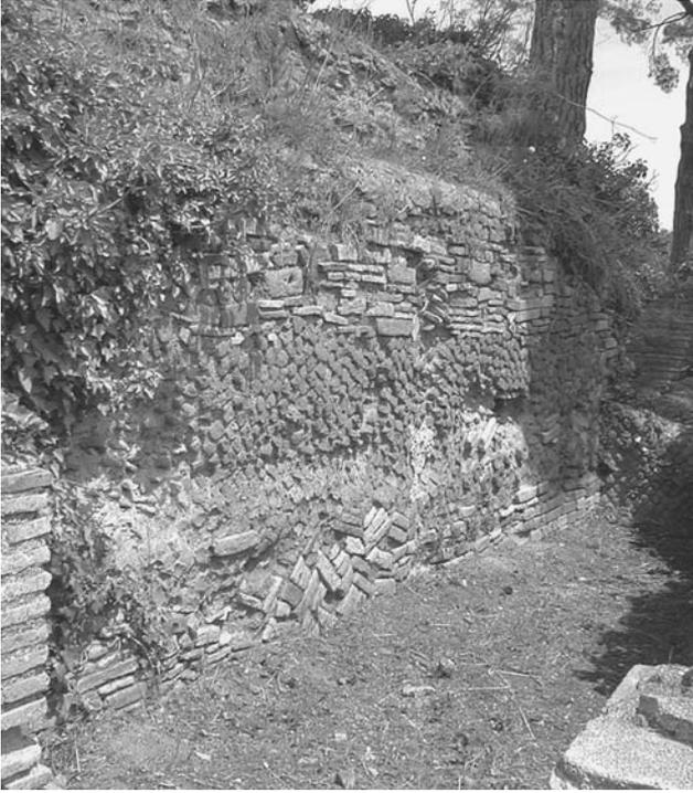
FIGURE 9.1. *Opus caementicium* wall with facing consisting in part of recycled pieces of pottery at Domus di Giove Fulminatore at Ostia. Photo: JTP.
