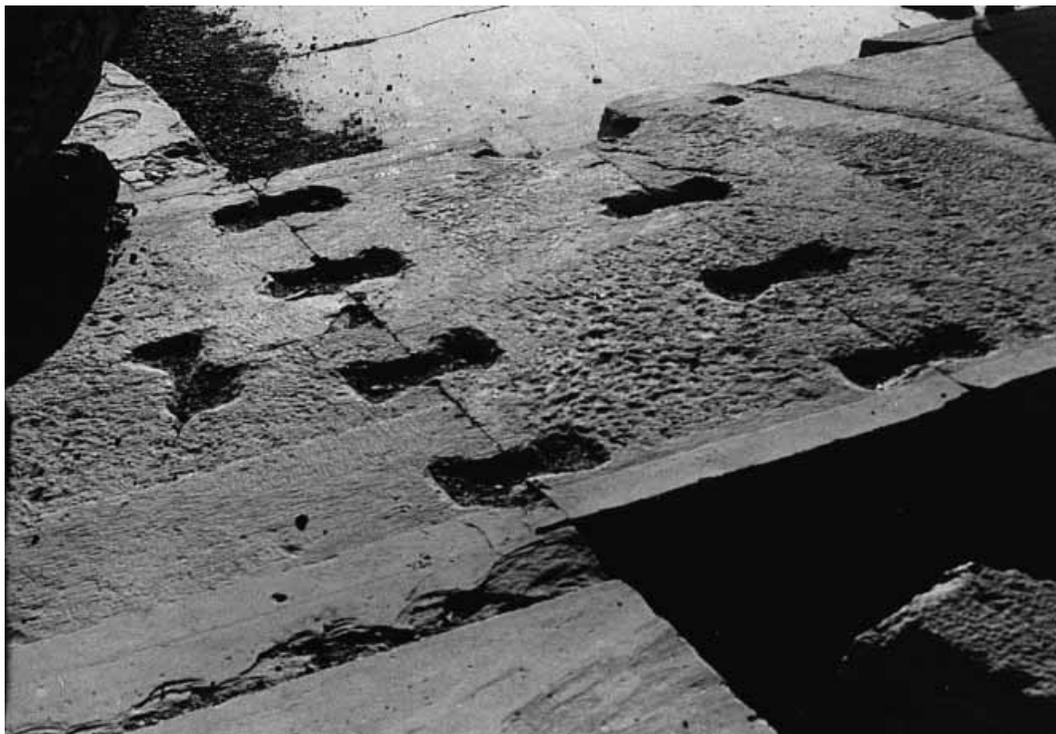
Plate 9.2 Detail of clamp holes in stone masonry at Pasargadae.
