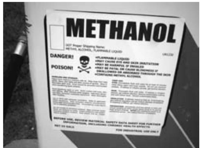
**FIGURE 11-22** Sign on methanol pump shows that methyl alcohol is a poison and can cause skin irritation and other personal injury. Methanol is used in industry as well as a fuel source.
