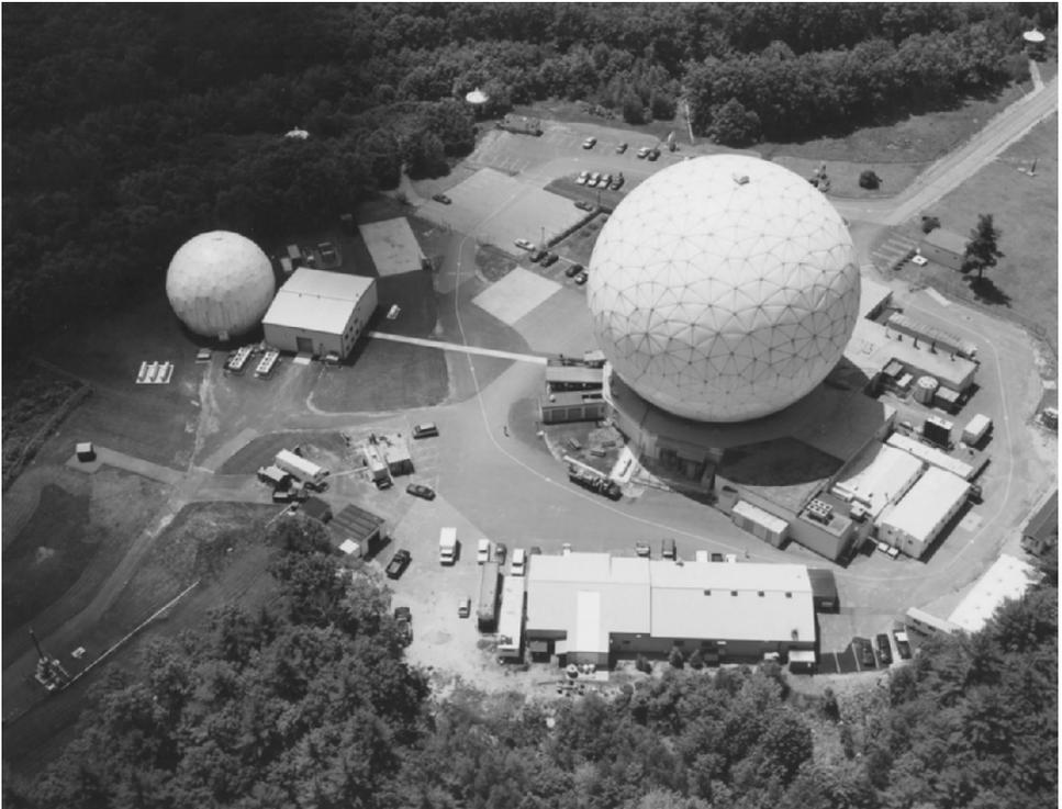
**Figure 3.6** Haystack and HAX radars located in Tyngsboro, MA. These radars collect 600 hours of orbital debris data each per year. They are NASA's primary source of data on centimeter-sized orbital debris. Courtesy NASA.
