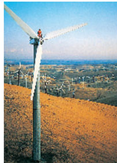
**Figure 25** Windmills work on the same basic principles as a power plant. Instead of steam turning a turbine, wind turns the rotors. **Describe** some of the advantages and disadvantages of using windmills.
