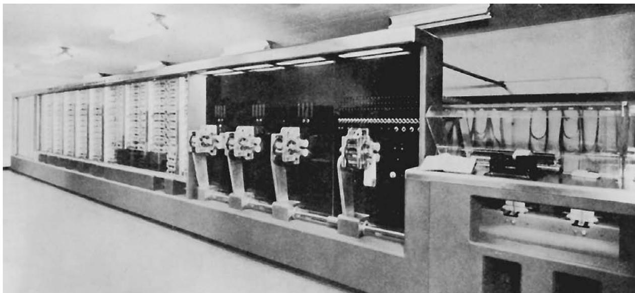
**Mark I computer, built in 1944 by Howard Aiken (1900–1973).** Aiken's calculator replaced mechanical components with electromagnetic ones and responded to instructions it was fed from punched cards. Aiken later introduced a computer science program to Harvard University, the first of its kind. THE LIBRARY OF CONGRESS
