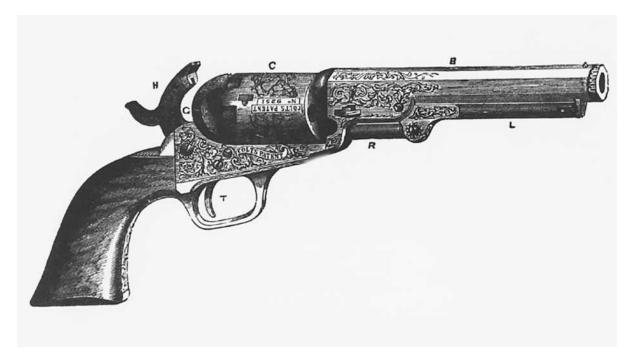
The original "Colt's Revolver," greatly increased firepower by enabling six shots to be fired before reloading. The revolving cartridge advanced the chambers each time the trigger was pulled.
