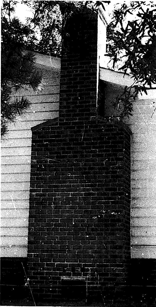
obstructions from the chimney and open wide the damper. An effective test material is tar paper, which creates more smoke as it burns than the fireplace will normally handle. Do not burn the test fire for a long period of time. A fire of lengthy duration must wait until the mortar is well cured.
