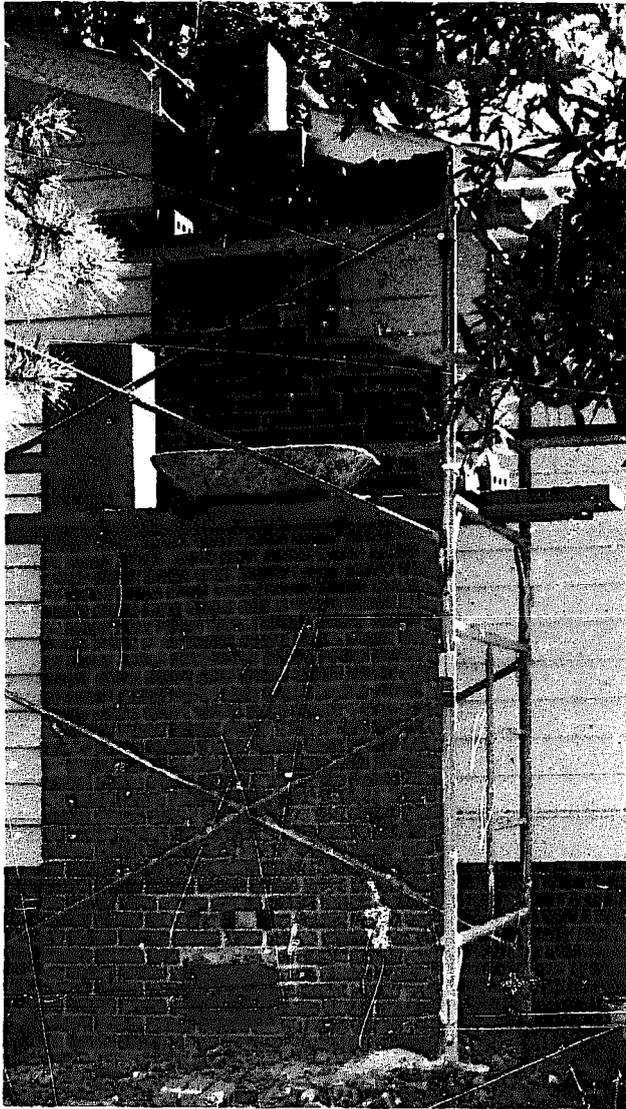
ing to complete the balance of the project. One worker on the ground can hand up materials to another above, who will set them in place. Plumb the sides of the liner. If the liner leans too far to one side, it will have to be shimmed or propped with a shard of brick, and any gaps will have to be filled with mortar. Reach inside the liner from its top to smooth the joint so that it will not collect soot.
