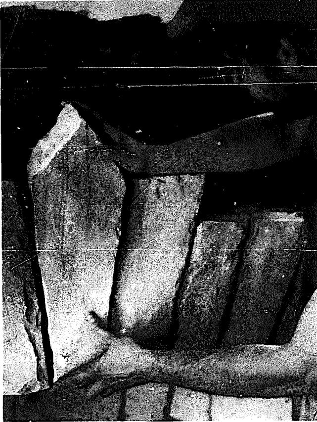
smoke will flow unobstructedly through the throat. If necessary, plaster a coating of mortar over the back side of the breast. When the breast is completed to the top of the firebox, the throat is complete. This is the time to build the smoke shelf.
