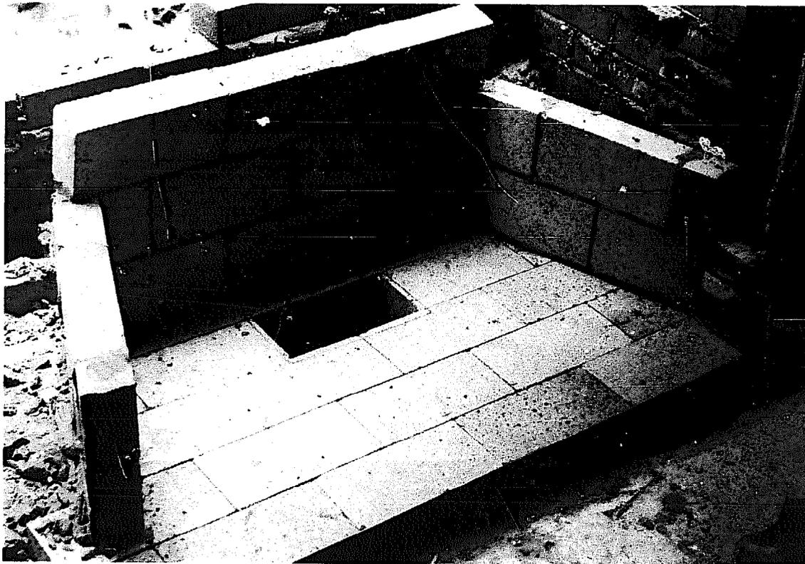
Ash dump/air supply should be farther forward.
